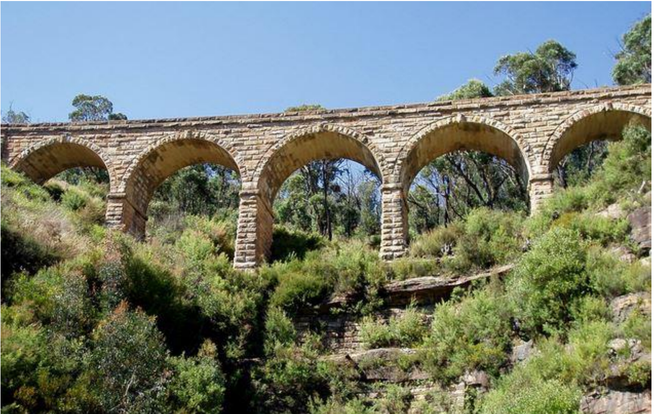
Zig Zag Railway Bridge, Lithgow LGA
