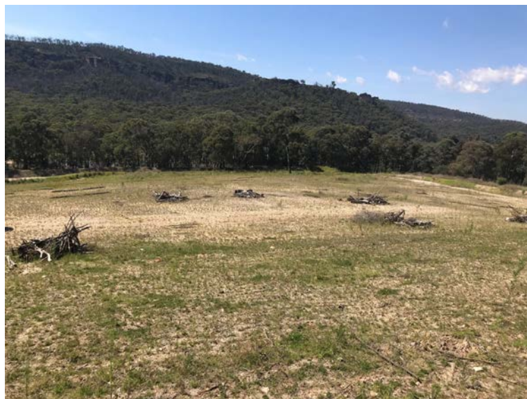
Cullen Bullen Landfill - rehabilitation
