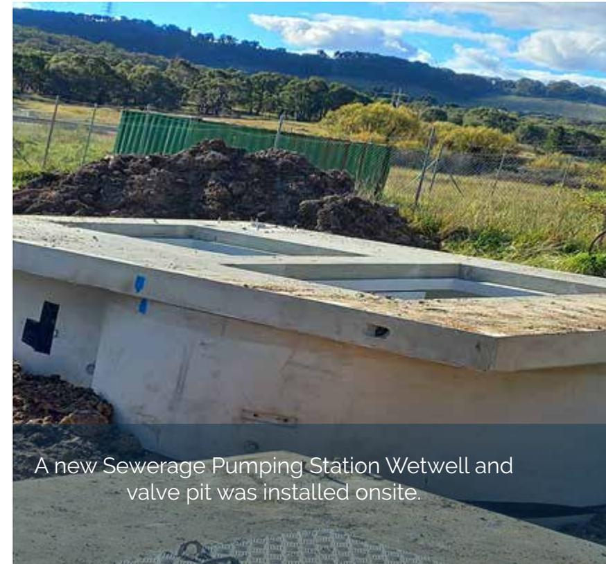
A new Sewerage Pumping Station Wetwell and valve pit was installed onsite.
