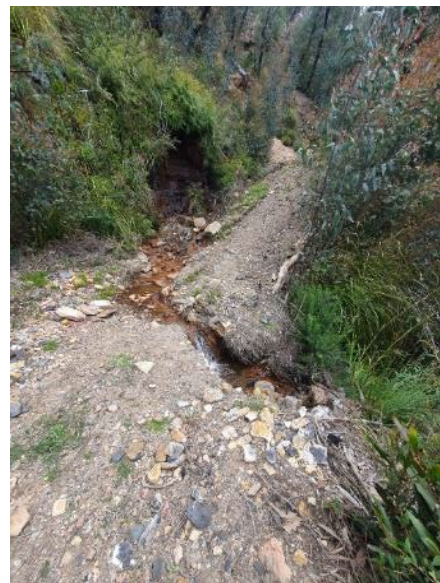
Plate 12 Waterway crossing the existing track
