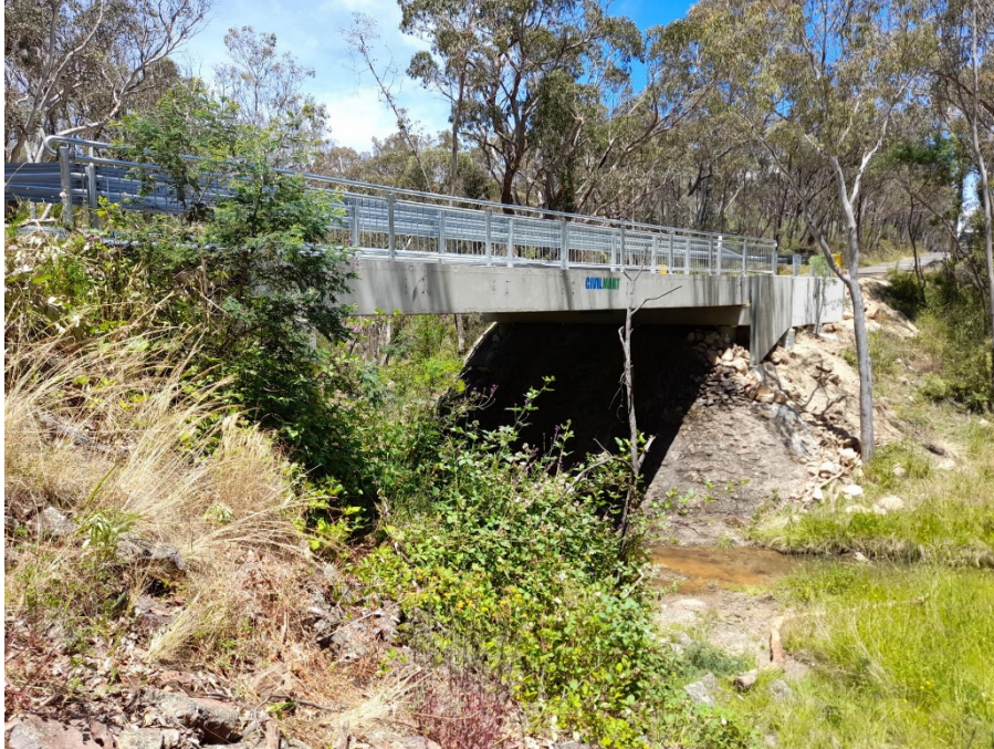
Photo: Completed Airly Bridge, Glen Davis
