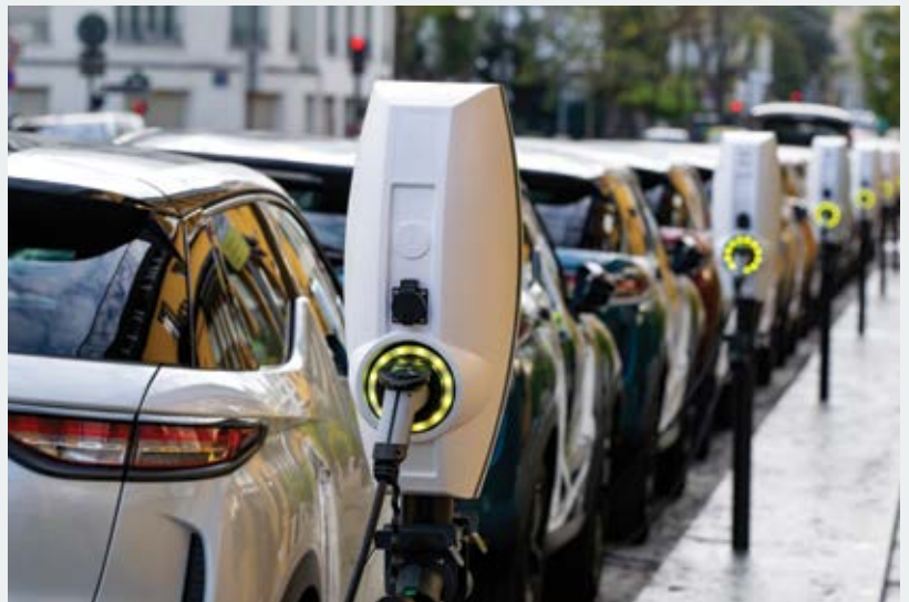
Figure 6 Example of multiple on-street Level 2 charge points for longer term stay periods 3
