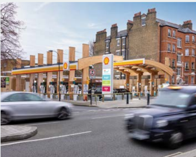
Figure 7: EV charging station similar to a petrol station (Fulham, London)
