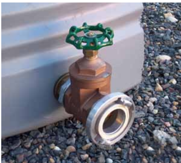
Figure 8. Gate Valve
