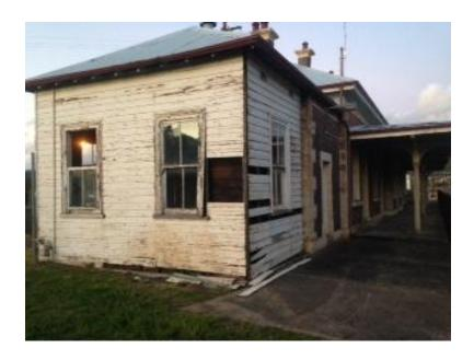
After the before mentioned works are carried out I would then propose to cut out severely fretted base course stones. New matching sandstone blocks would be laid on 20kg/m² lead flashings to reduce rising damp issues.
