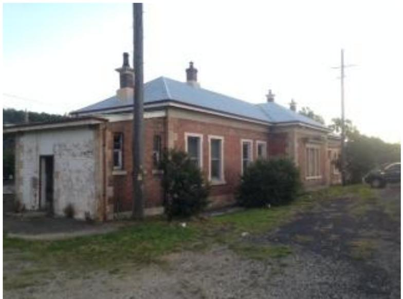
The Long term objective would be to remove all concrete and bitumen paving to ground level external to building and also remove all concrete slab floors within the building. It seems where the original timber floors have rotted out they have been replaced with concrete.
