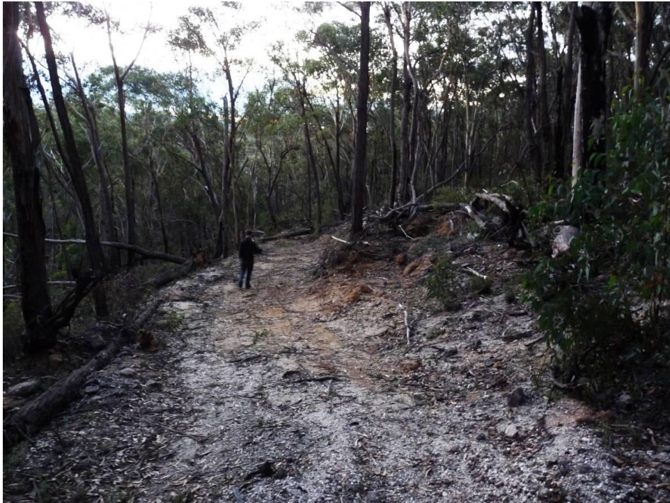
Plate 6: Significant earthworks and clearing is evident along the right hand fork.
