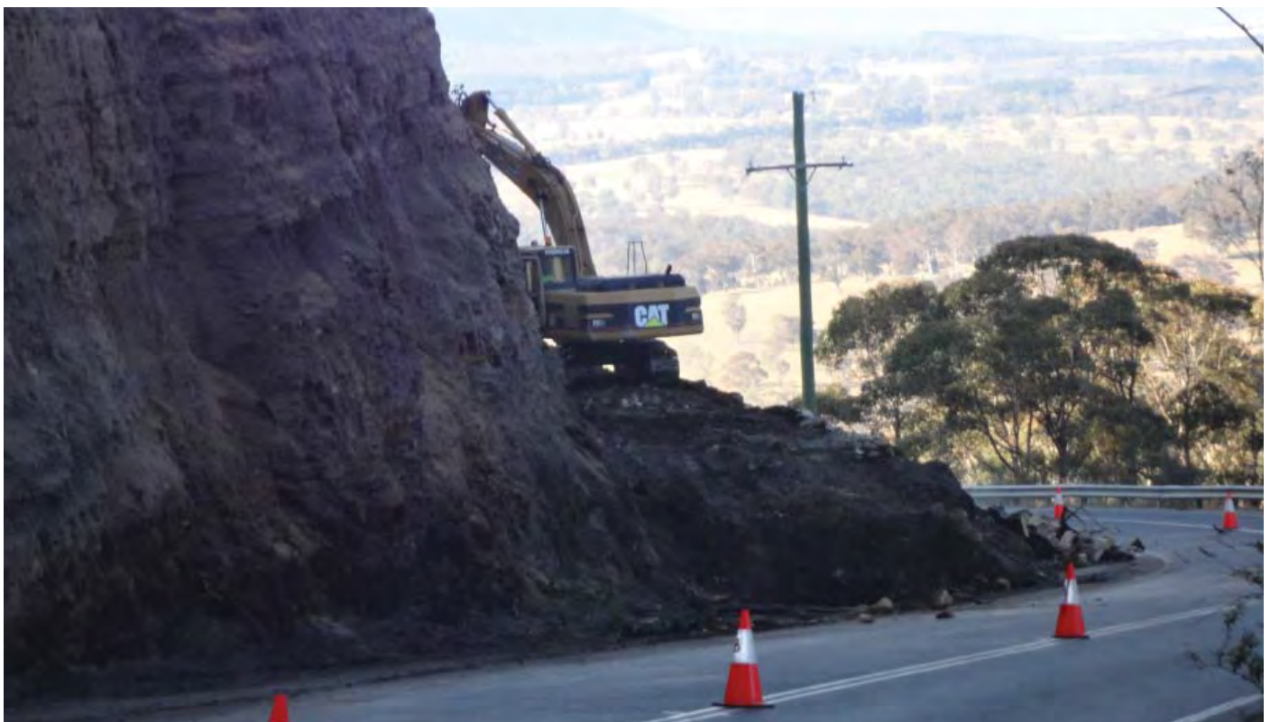
Road Safety Works being undertaken on Browns Gap.
