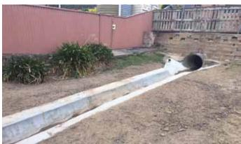
Pictured: Completed stormwater drainage works at La Salle Academy.
