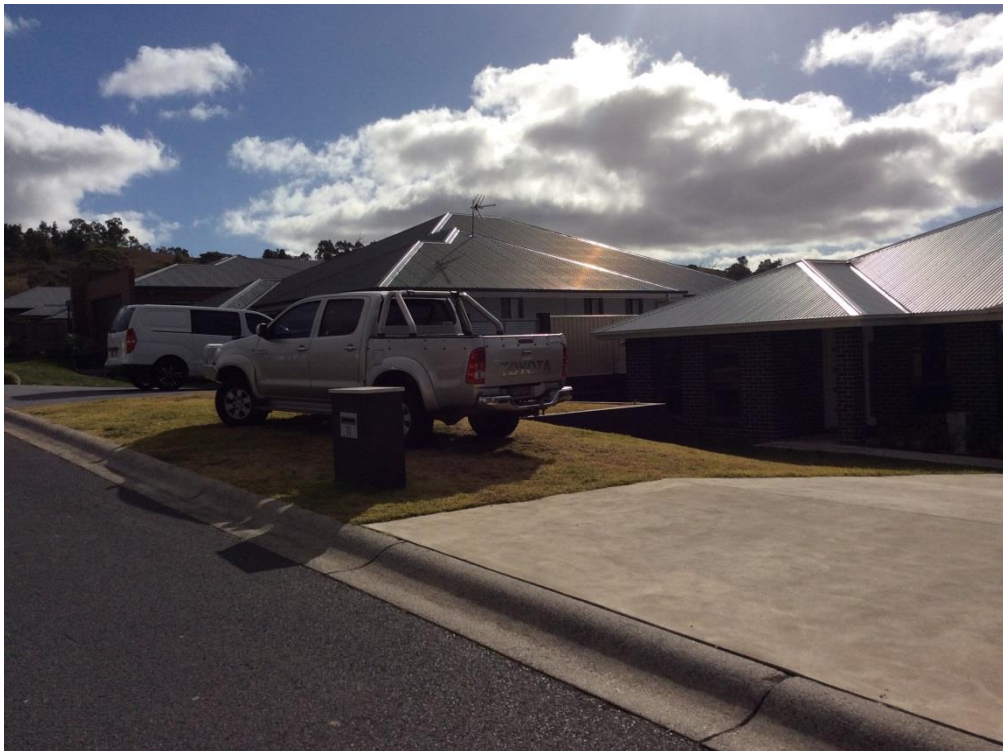
View to the south west and impact of SFH/flue on neighbouring property to the south (No. 13)
