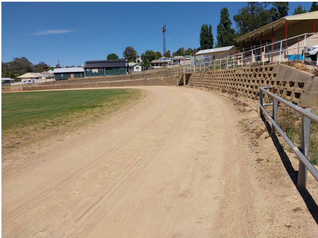
Figure 2 – Existing Arena Retaining Walls at Kremer Park Proposed Development
