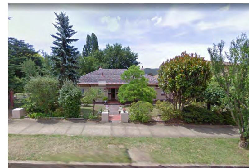
VIEW 01 - NO 4 CHURCH STREET
