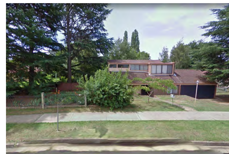
VIEW 01 - NO 6 CHURCH STREET
