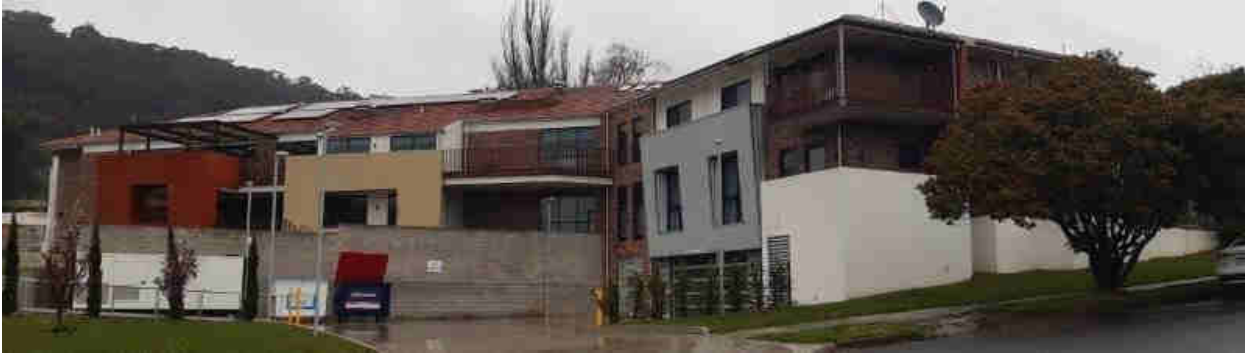
View of Building A from internal parking area (looking north-west)
