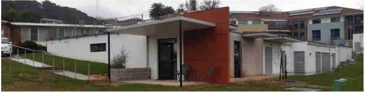
View of original Coinda buildings from Maple Crescent (looking south-west)
