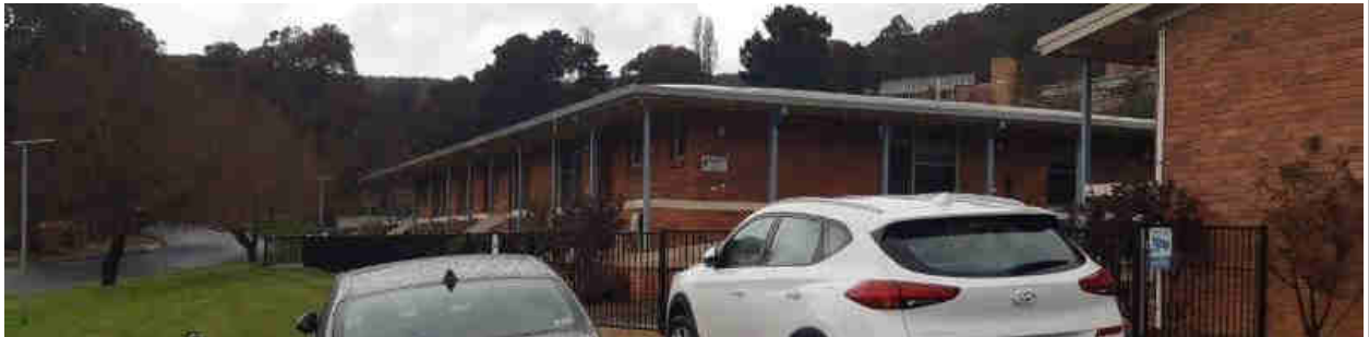
View of Madden House from Maple Crescent (looking south-west)
