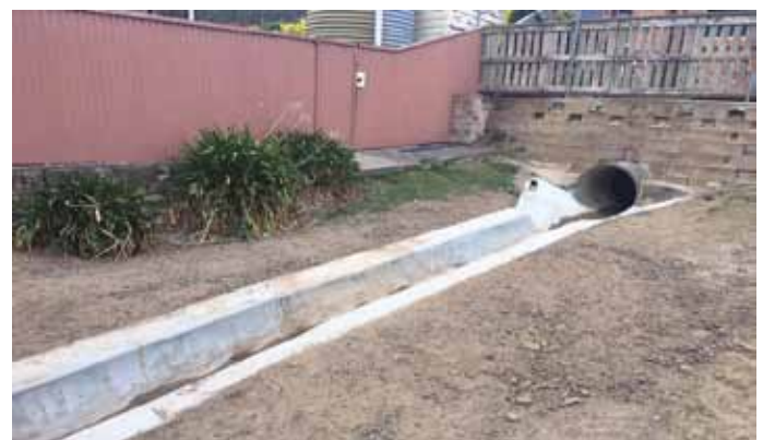
Pictured: Completed stormwater drainage works at La Salle Academy.
