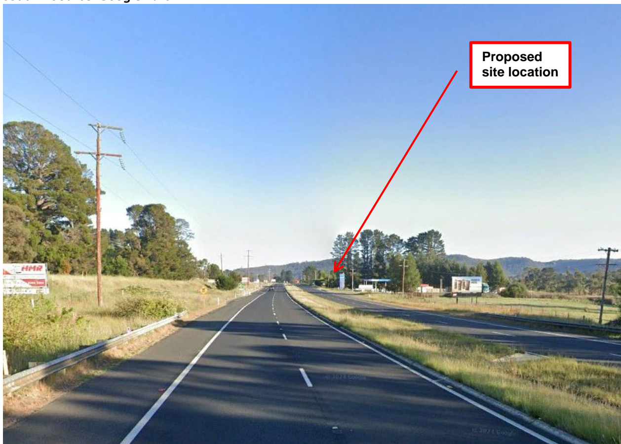
Image 11: View towards the proposed site location from Great Western highway, approximately 290m south – Source: Google Earth
