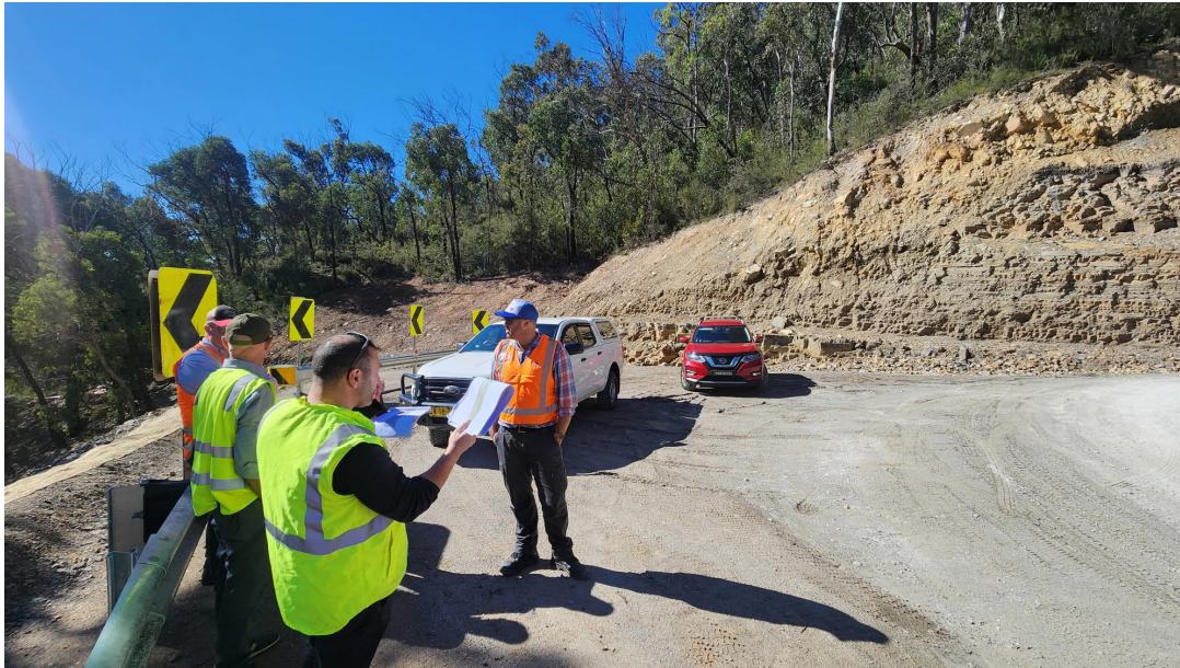
Site Visit 14 May 2024: with CJC Management, Wassabi Group and WSP
