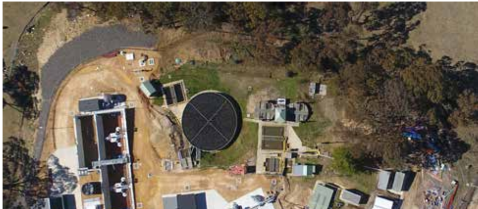
Portland Sewerage Treatment Plant
