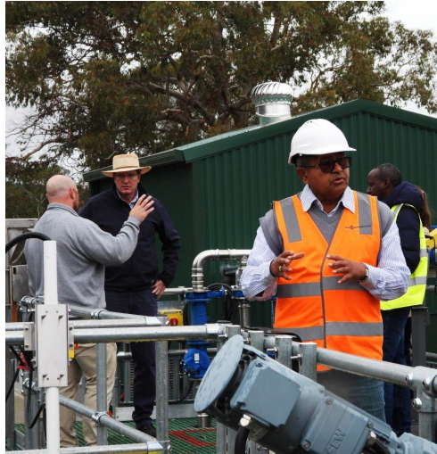
MAY Opening of the Cullen Bullen Sewerage Plant
