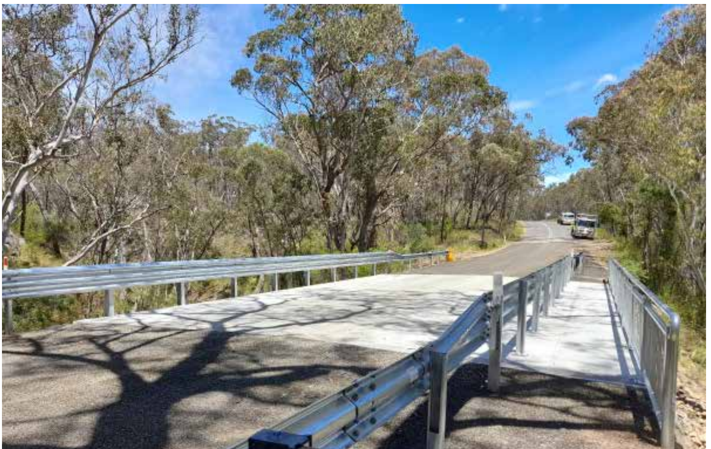
Airly Bridge, Glen Davis Road, Capertee Valley complete with pedestrian access for bird watching.
