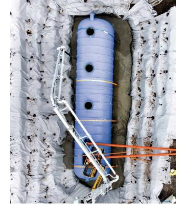
Guaranteed hydrocarbon spill capture in all flow and spill conditions. Spillceptor is a full retention separator that treats all flows.
