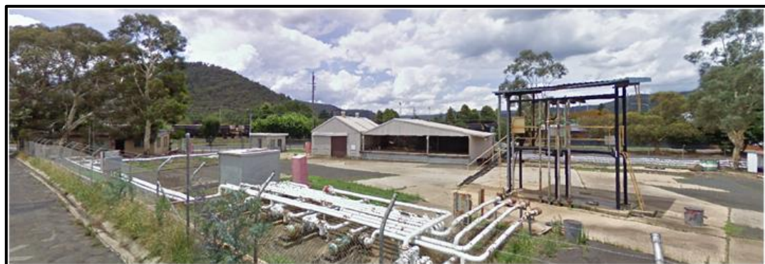
Figure 9: View of part of old fuel depot that is the subject site for the service station development
