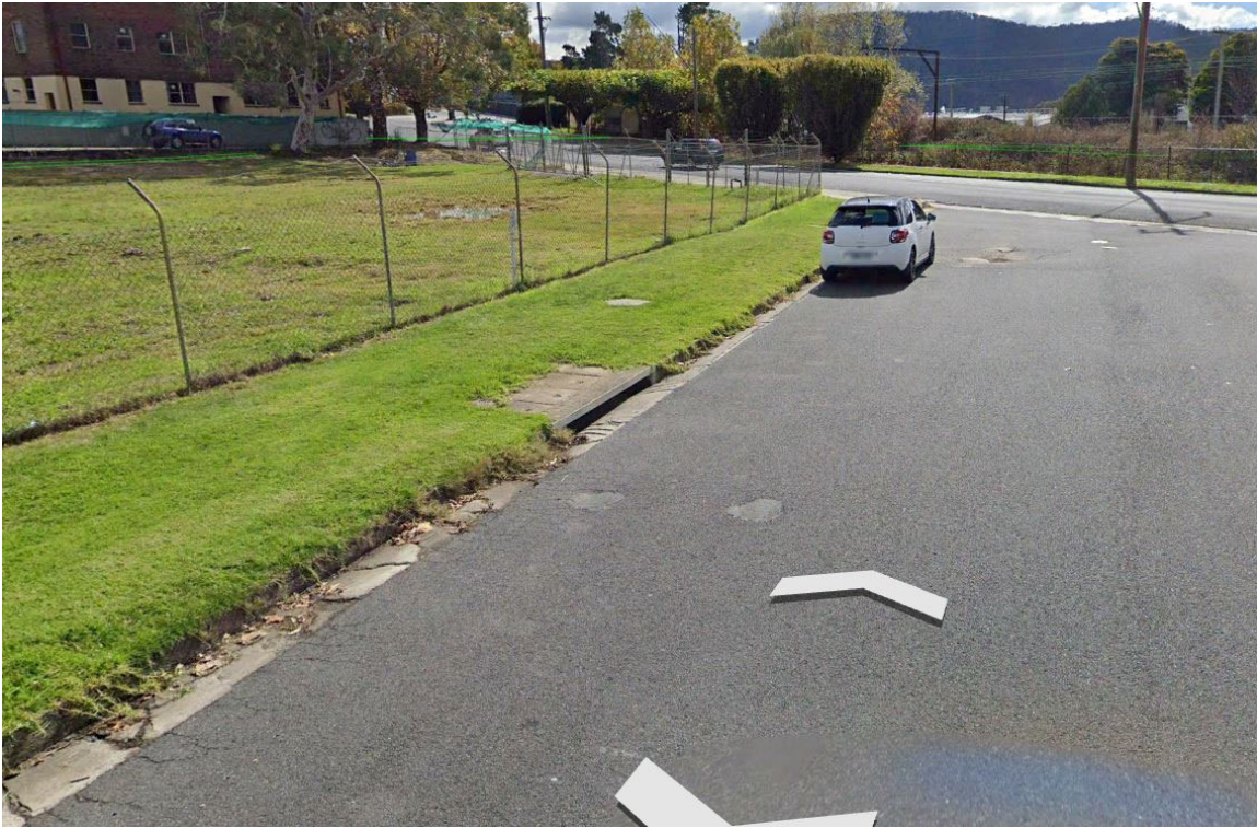
Figure 2: Existing Stormwater Pit in Endfield Street
