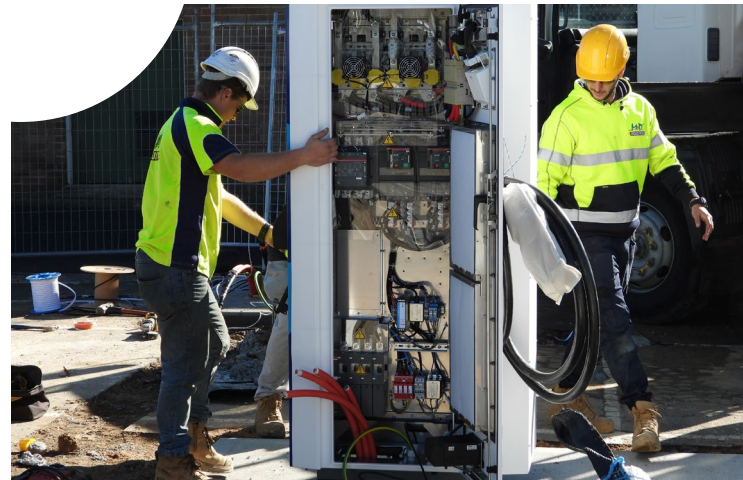
Installation of NRMA charges at Eskbank Street Park
