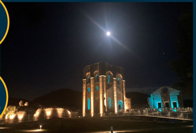
Light Installations at Blast Furnace
