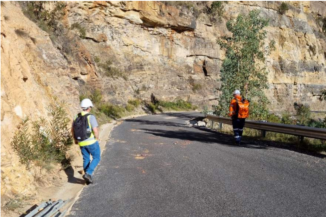
Figure 1 Example of small gravel sized rockfalls observed on road, February 2025.
