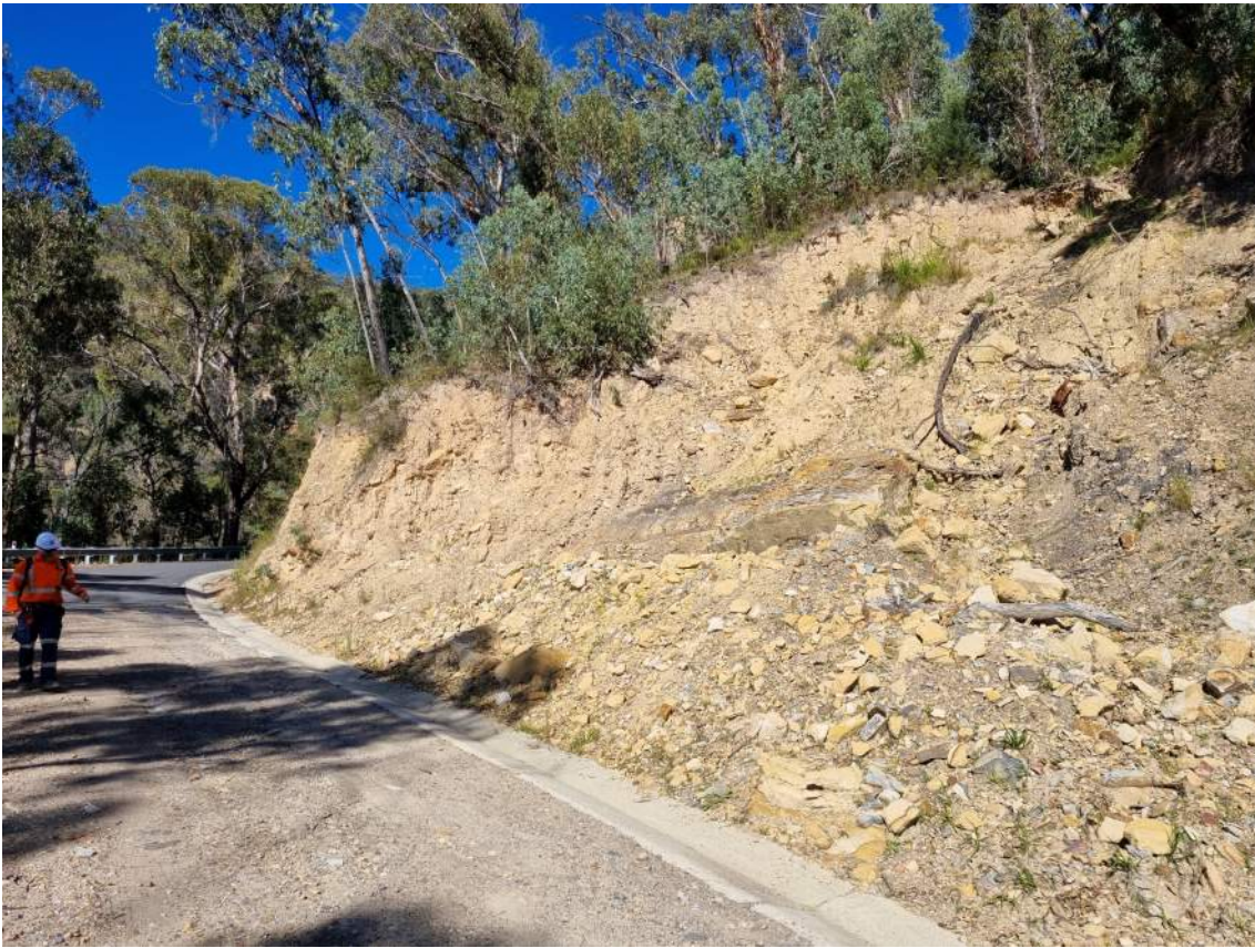
Figure 7 Example of upslope batter failure in colluvium, talus and weathered bedrock along of lower section of Wolgan Road.
