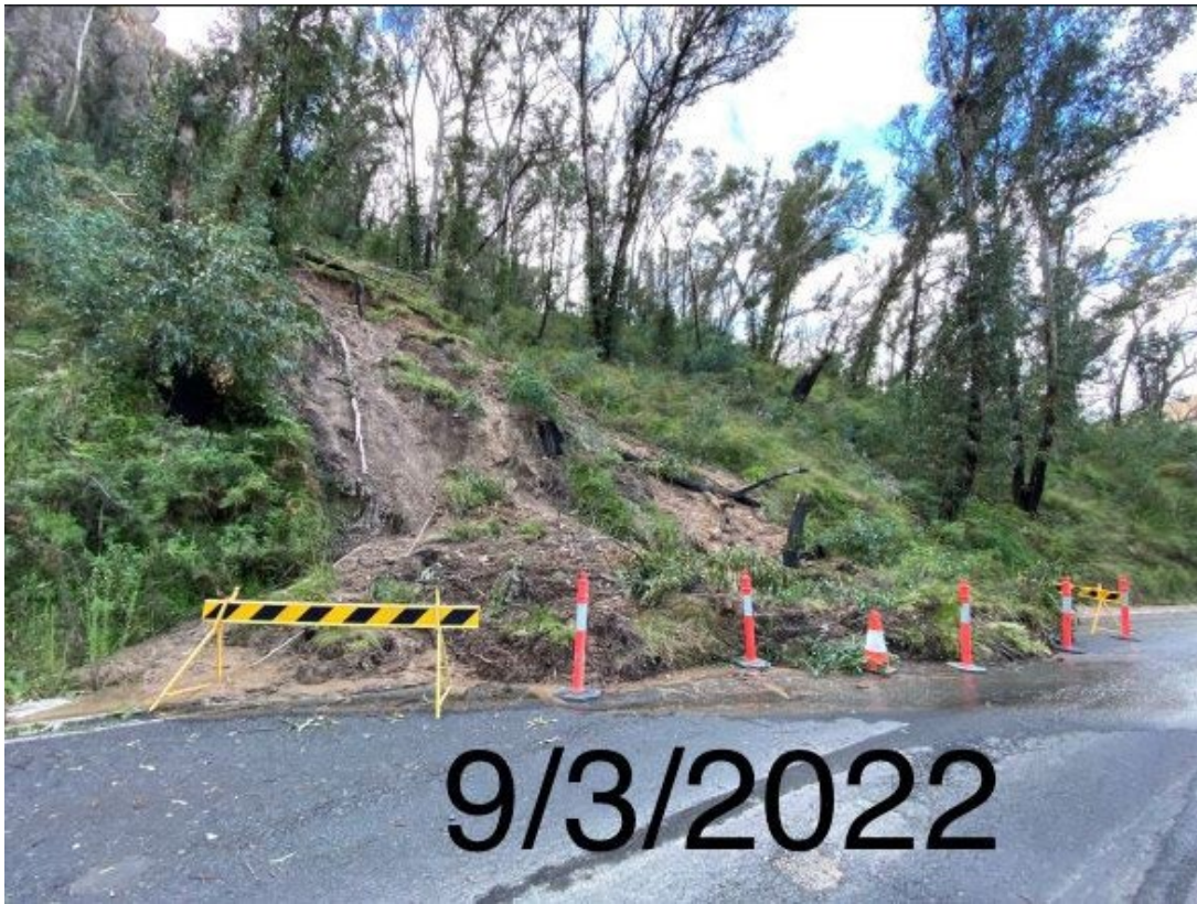
Event 71 - Resident's photo showing landslide, taken 09/03/2022.
