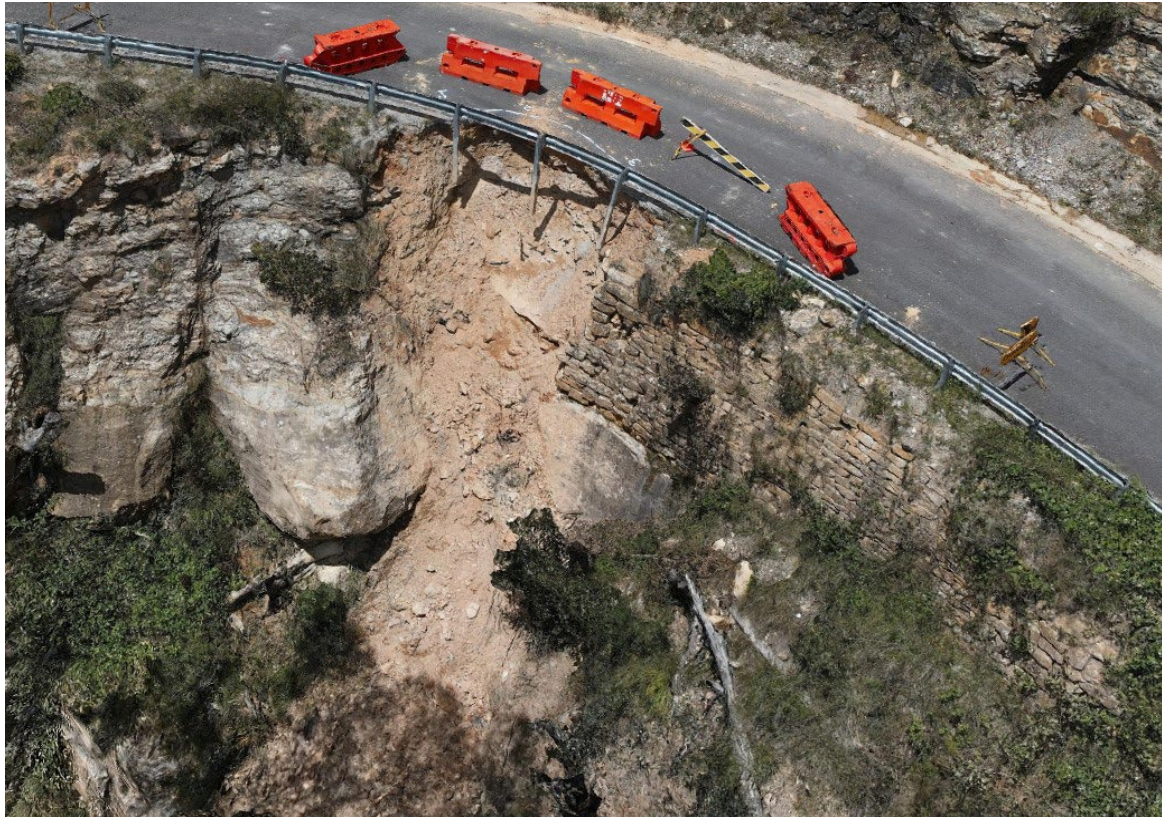
Event 68 - Aerial Photogrammetry showing embankment failure, captured 13/12/2021.
