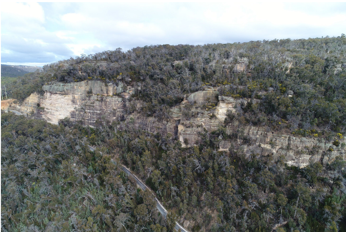
Figure 12 View to south of cliffs and colluvial slopes in Domain 2. Domain 1 cliffs on left at top of The Gap.
