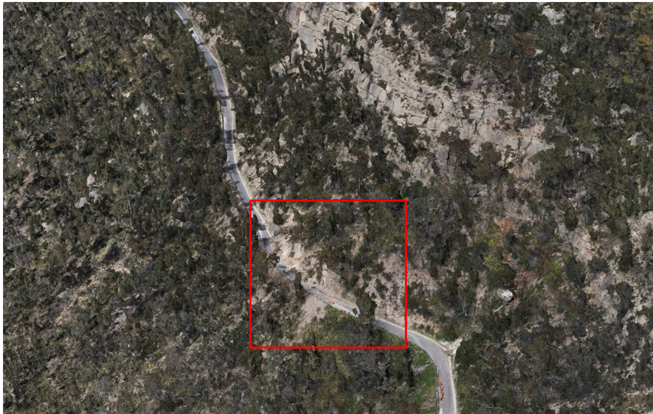
Event 85 - Aerial photogrammetry showing landslide, captured 15/11/2022.
