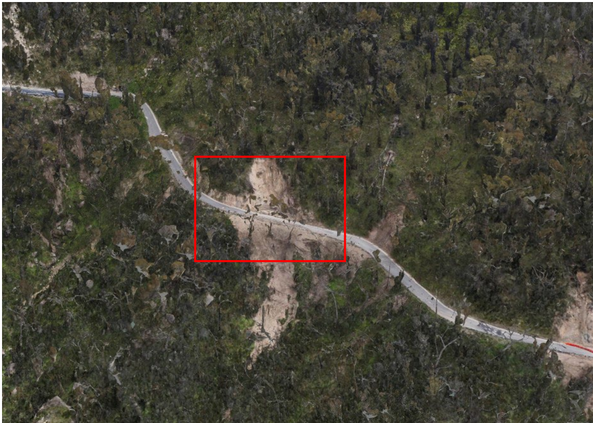
Event 76 - Aerial photogrammetry showing landslide, captured on 15/11/2022.
