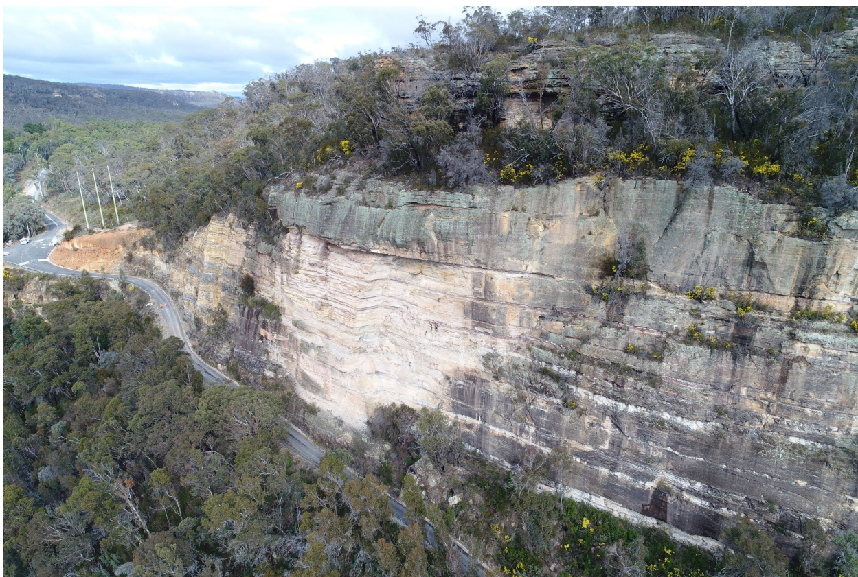
Figure 9 View to south of cliff and rock cuttings in Domain 1.
