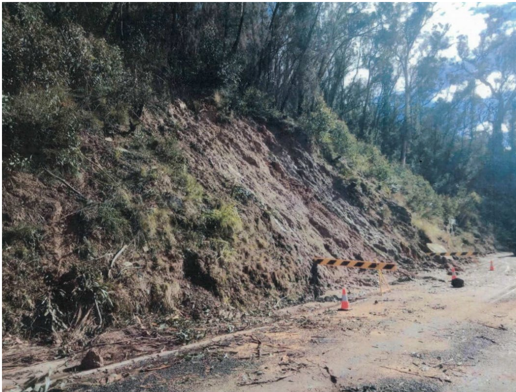
Event 63 - Resident's photo showing remnants of rockfall debris, taken 12/03/2021.
