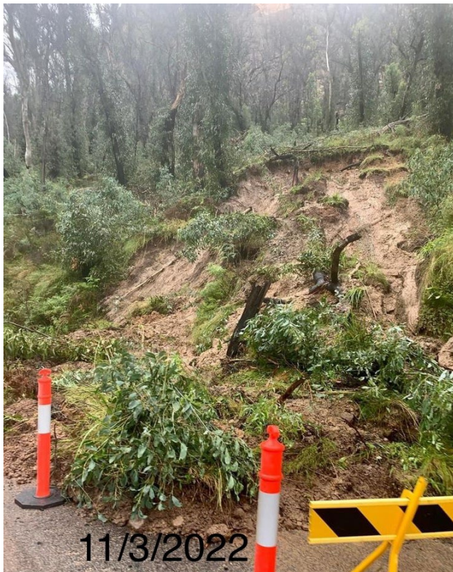
Event 71 - Resident's photo showing landslide, taken 11/03/2022.
