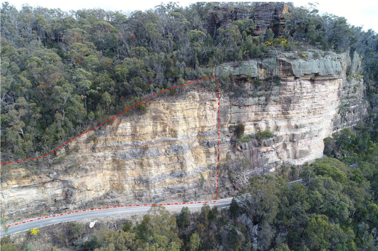
Figure 7 Drone / UAV photograph acquired by GHD showing (red outline) the approximate extent of the cliff removed / widened by blasting in 1962/1963.
