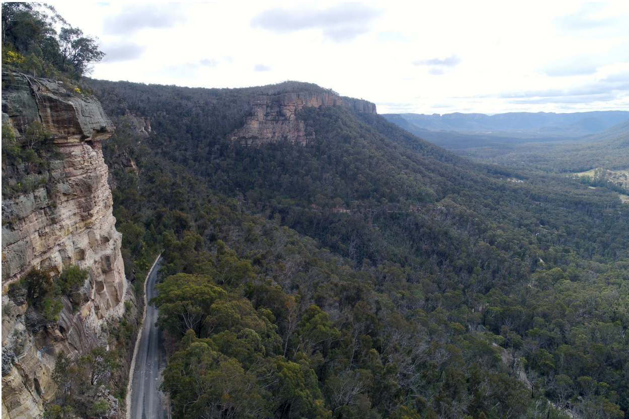
Figure 2 View of Wolgan Road looking north. Donkey Steps track on right.
