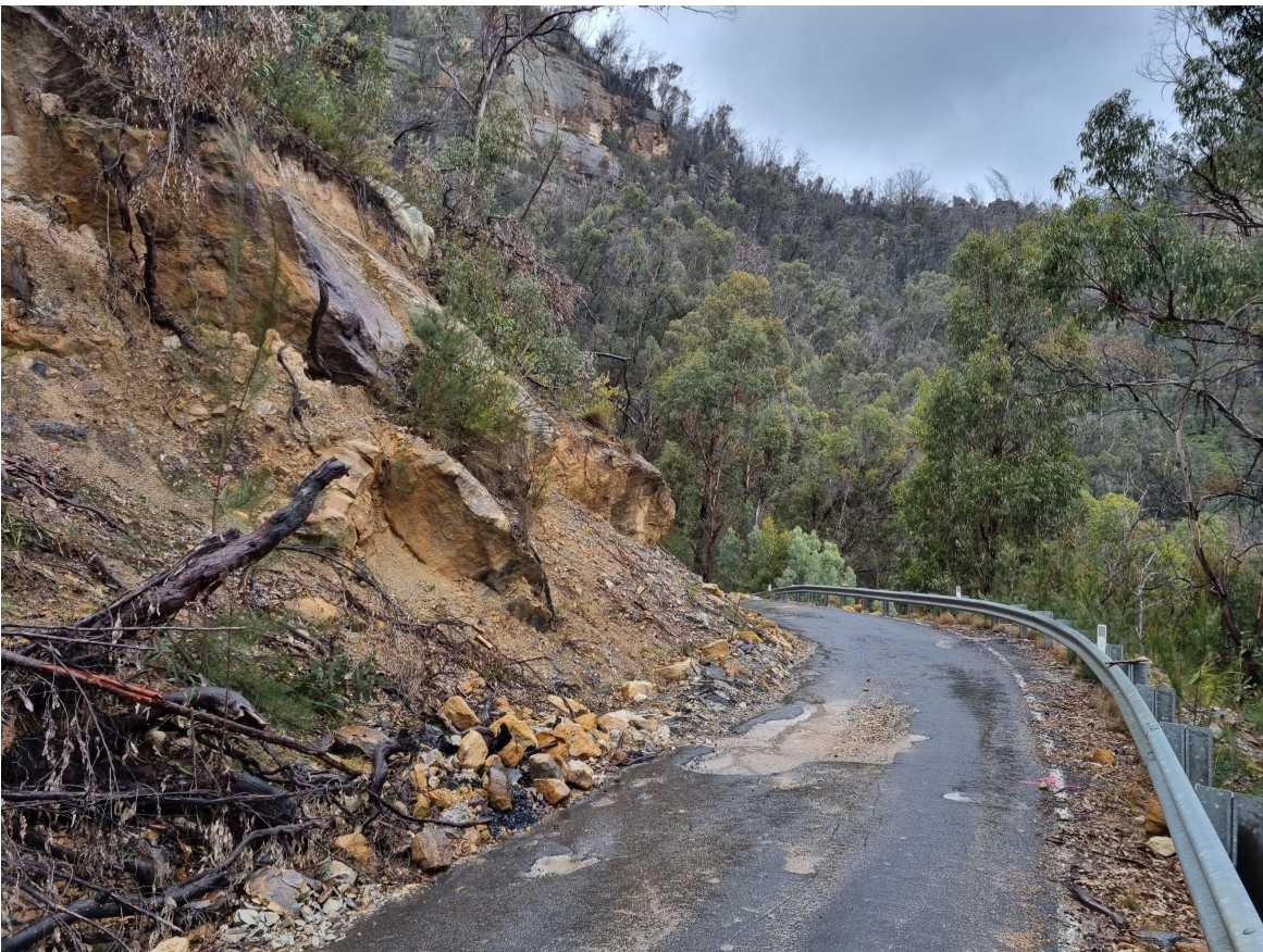
Figure 14 Toe of landslide in colluvium
