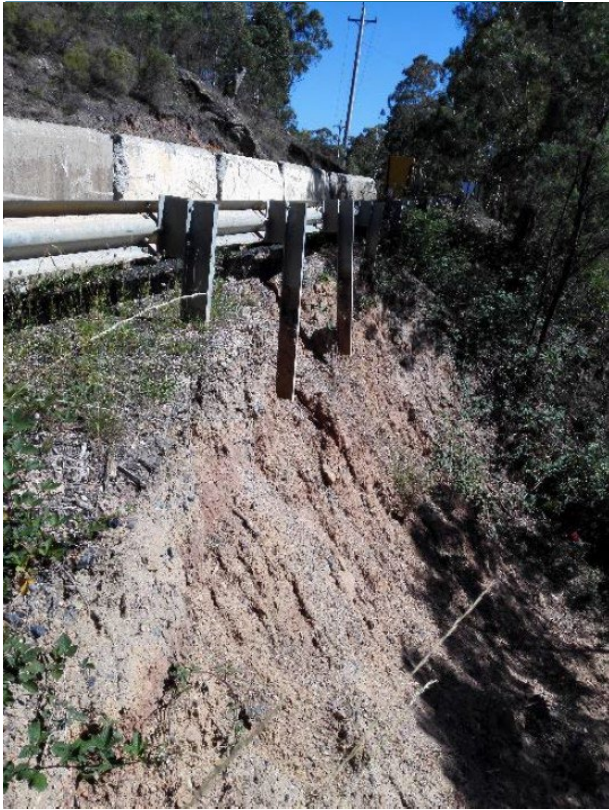
Event 52 - Photo of Embankment Failure, taken from Golder remediation report, 2018.
