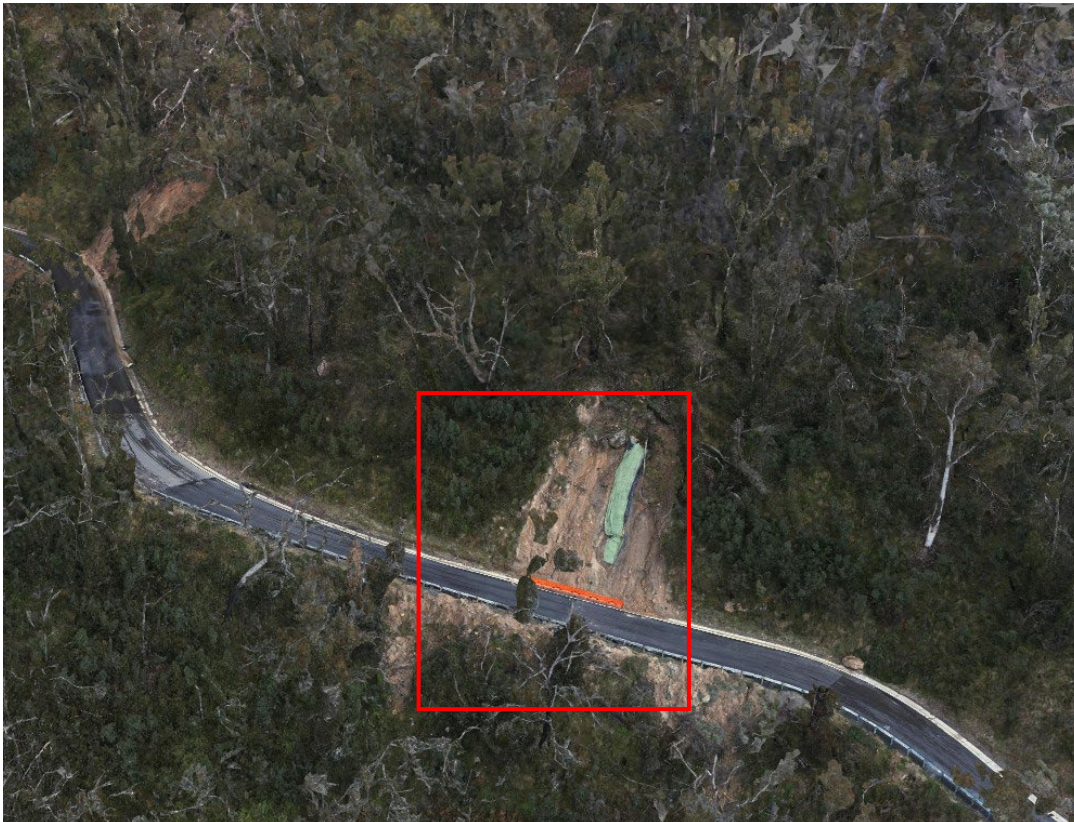
Event 74 - Aerial photogrammetry showing landslide, captured on 29/08/2022.
