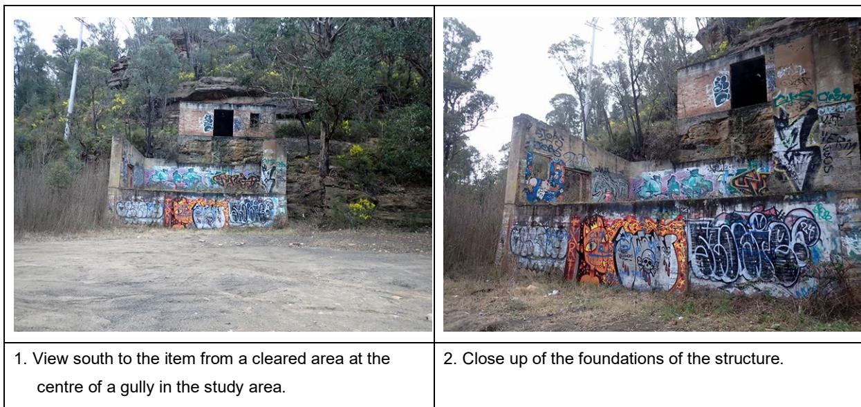
Figure 4-3: View of HS02: the Dobbs Drift.
