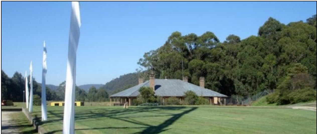
Figure 3-6: View towards the State Mine office building and the old horse paddock behind that is proposed to be used as a car parking area.
