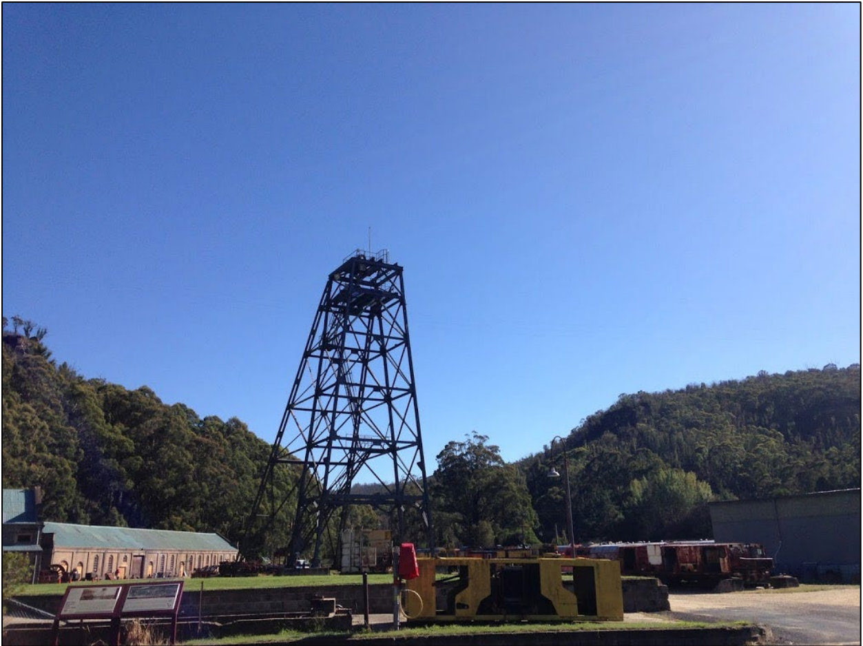
Figure 3-9: Views towards the restored 1923 poppet head.
