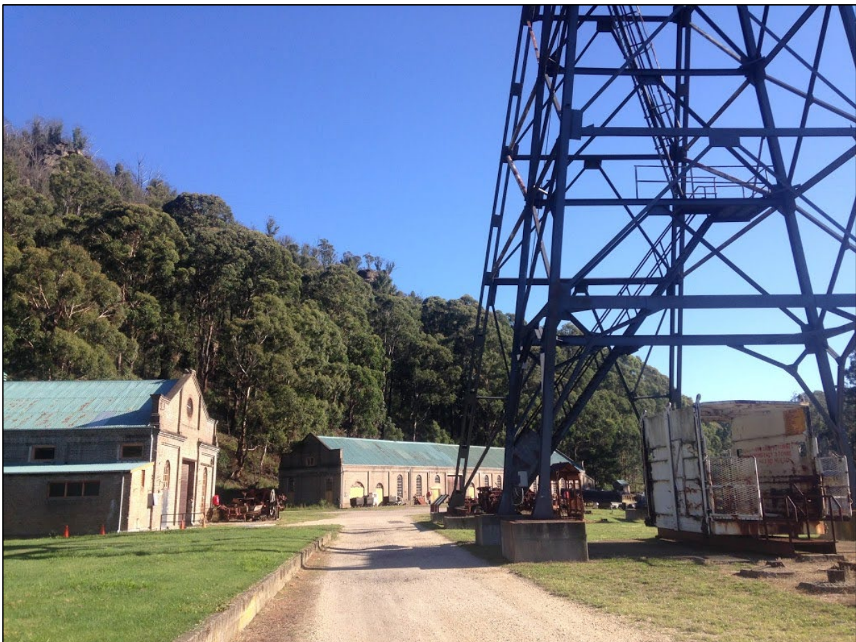
Figure 3-12: View towards the workshop and stores building.
