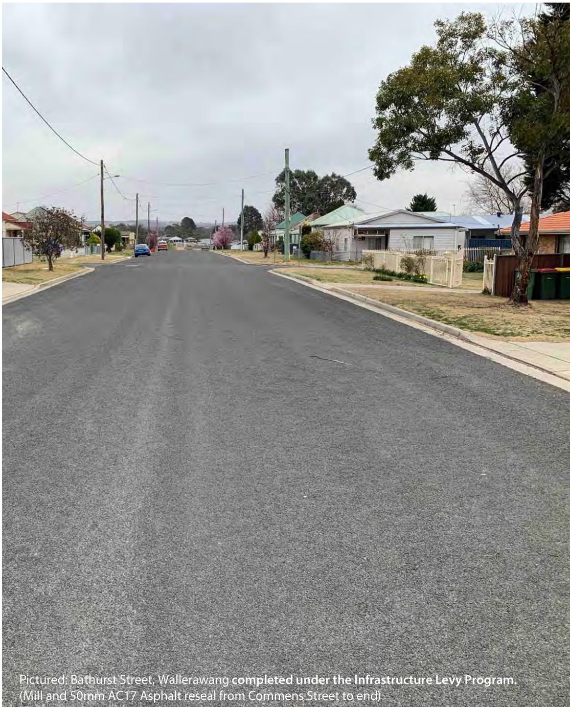
Pictured: Bathurst Street, Wallerawang completed under the Infrastructure Levy Program. (Mill and 50mm AC17 Asphalt reseal from Commens Street to end)
