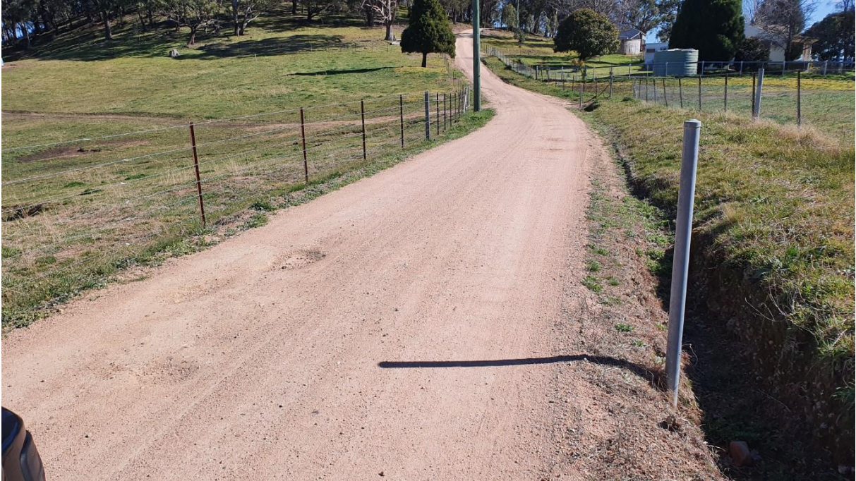
Approximate Ch 400 looking North with several potholes.
