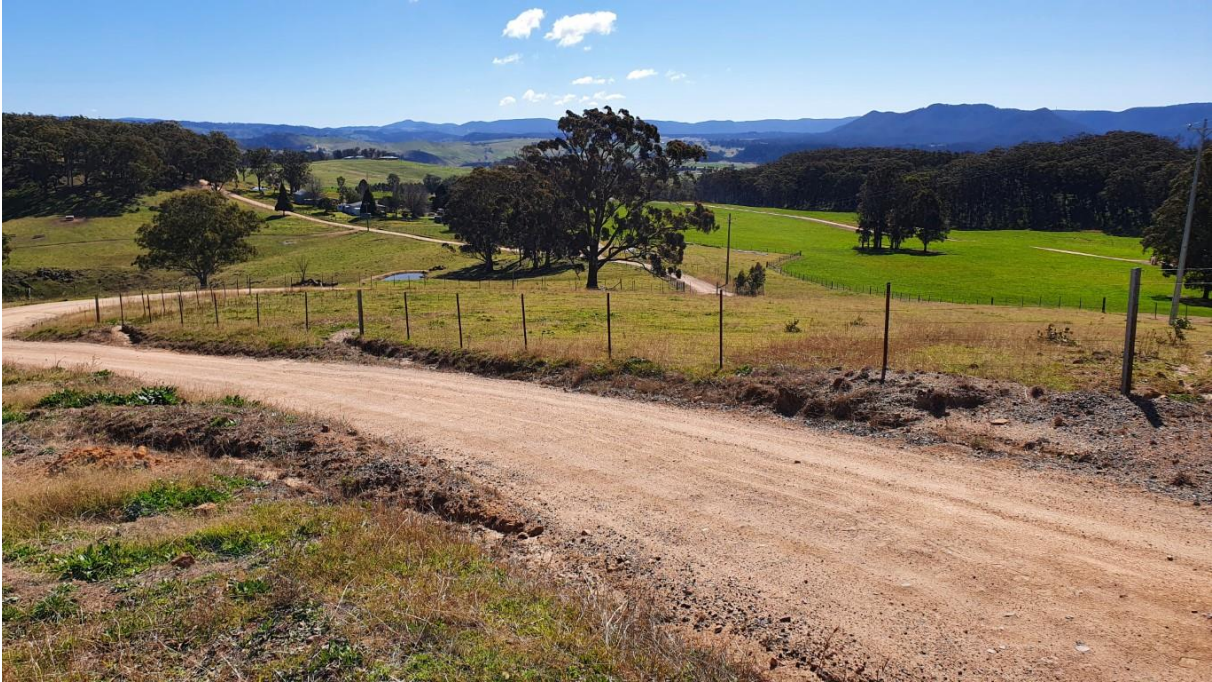
Approximate Ch 40 looking North with minor corrugations. Good regular mitre drains.
