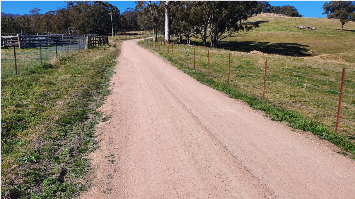
Approximate Ch 400 looking South with minor corrugations. Stable verges and drains.
