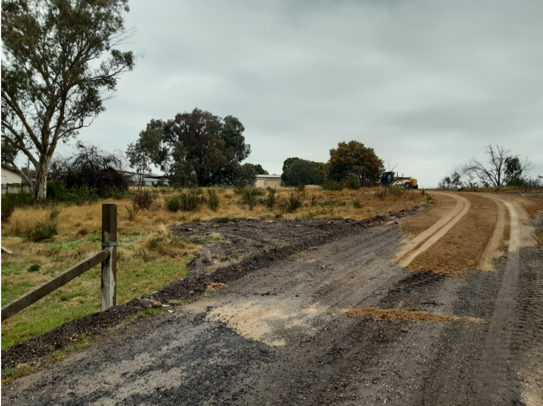
General site conditions (existing) near the top of the access handle (facing south west)
