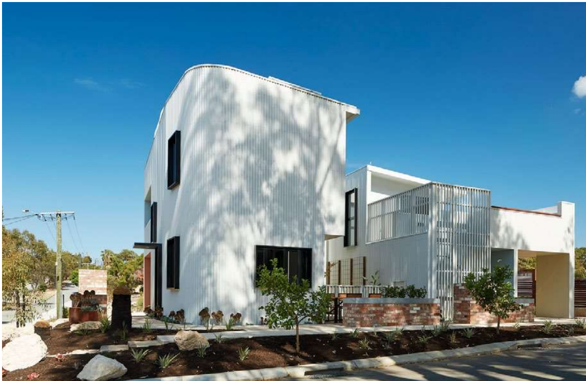
Figure 2-30 Manor House - 3 dwellings
