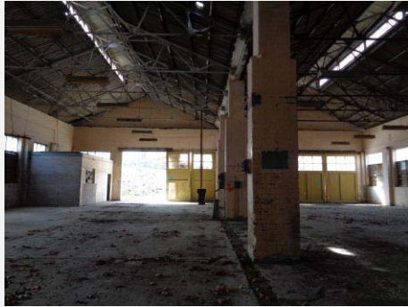
Plate 84: Interior showing Fitting and Machine Shop room (eastern room).
