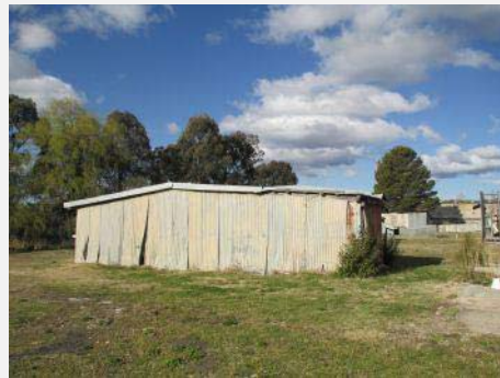
Plate 171: Area north of Cottages showing outbuildings.
