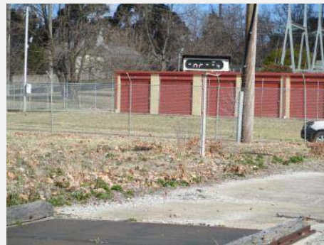
Plate 108: Part west elevation showing original building with some discolouration on brickwork caused by moss.
