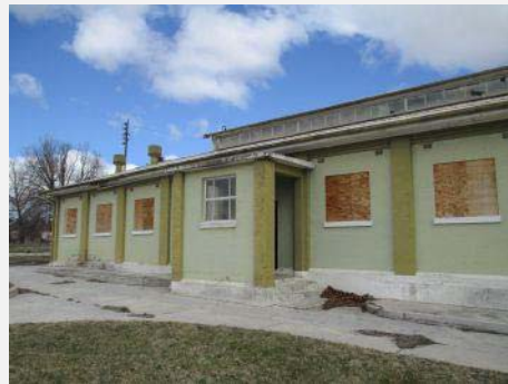
Plate 121: Shower and Bath house part north elevation.
