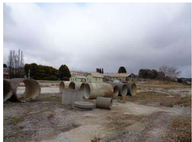
Plate 21: View of Ambulance Station, Workshop (Small store) and Annex building looking south west from The Powerhouse building.
