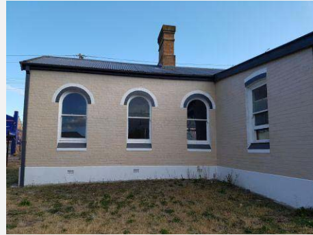
Plate 216: Casino building part north elevation.
