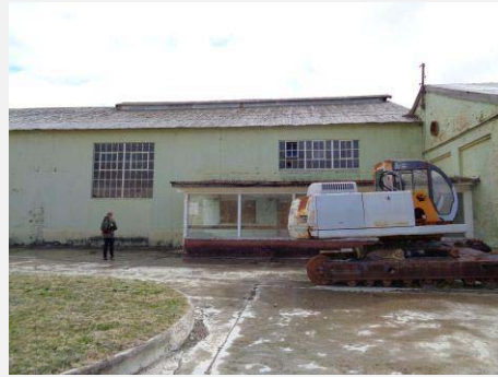
Plate 50: Boilerhouse part south elevation with later addition (single storey building in front).
