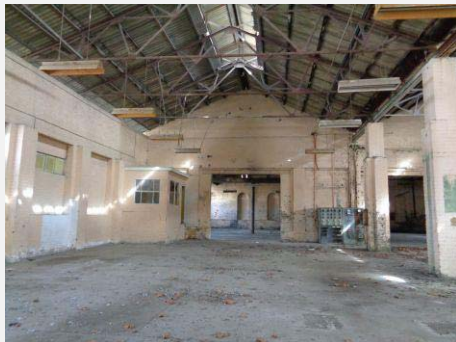
Plate 80: Interior showing Fitting and Machine Shop room (eastern room).
