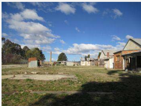
Plate 172: View of rear of Cottages looking east showing outbuildings.
