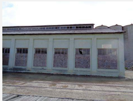
Plate 79: Boilermaker's / Blacksmiths Shop part south elevation.
