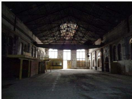
Plate 14: Interior looking south showing exposed trusses.
