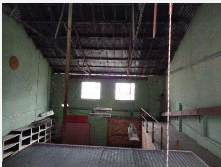
Plate 71: Interior of Eastern room showing view from mezzanine level.
