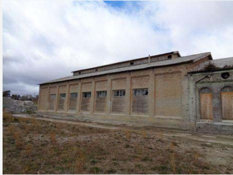
Plate 76: Boilermaker's / Blacksmiths Shop part north elevation.
