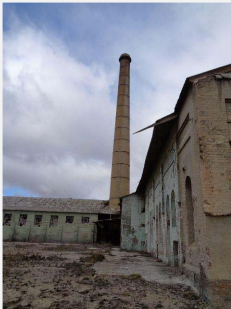
Plate 53: Part north elevation of Chimney and Boilerhouse (left).
