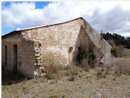
Plate 224: North east view.
