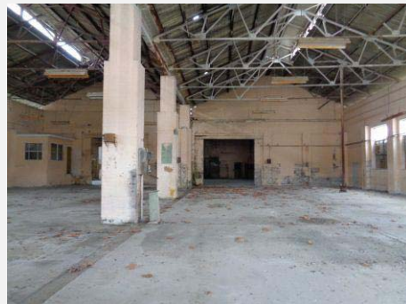
Plate 81: Interior showing Fitting and Machine Shop room (eastern room).
