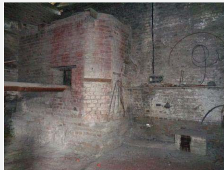
Plate 229: Interior main room showing remnant limewash.
