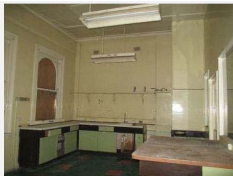
Plate 145: Interior showing kitchen area with timber joinery and linoleum flooring.
