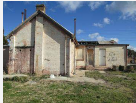
Plate 163: Cottages 7 & 8 north elevation.
