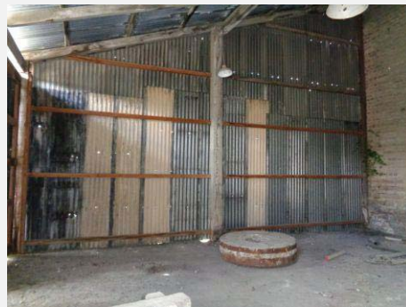
Plate 225: Interior north west room.
