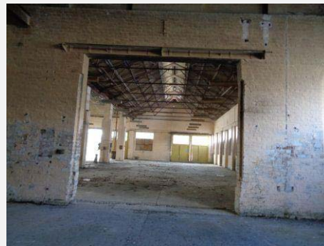
Plate 95: Interior showing Boilermaker's / Blacksmith's Shop.
