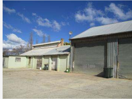
Plate 182: Part north elevation showing metal shed to the west.
