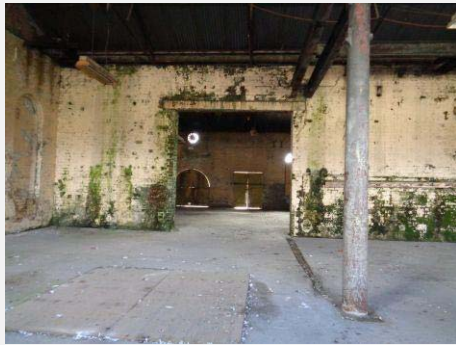
Plate 92: Interior showing Boilermaker's / Blacksmith's Shop.
