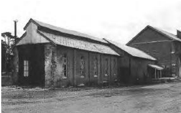
Plate 11: 1993 Loco shed (now demolished) (Source: Fenwick 1993)
