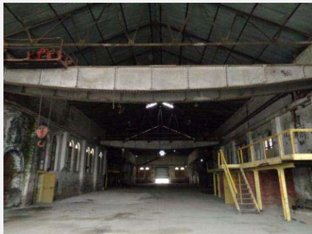
Plate 12: Interior looking north showing gantry.
