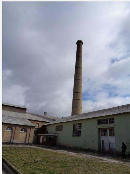
Plate 54: Part south elevation of Boilerhouse and Chimney (right).
