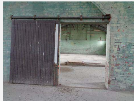
Plate 64: Interior of Central room showing sliding door leading to Western room.
