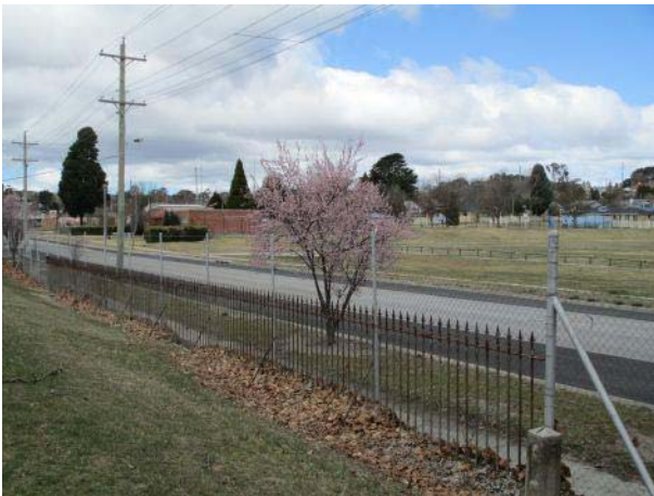
Plate 18: View of Williwa Street looking south east showing southern boundary to site and remnant cast iron fencing.
