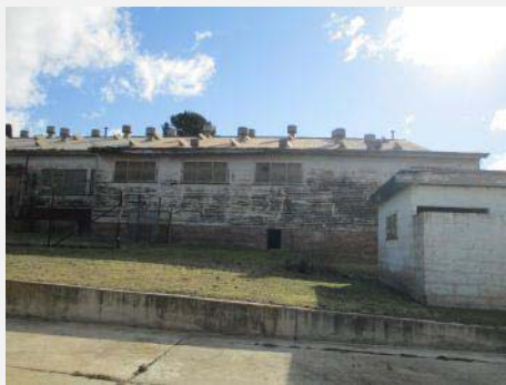
Plate 196: Part east elevation showing masonry structure to the right.
