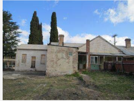
Plate 159: Part west elevation showing original building (left) additions (right with lighter brickwork).
