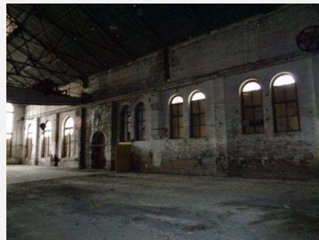
Plate 15: Interior looking west showing boarded windows.
