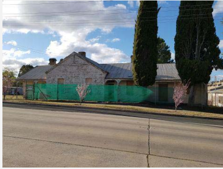
Plate 158: Cottages 1 & 2 south elevation.
