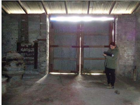
Plate 230: Interior main room showing corrugated iron doors.
