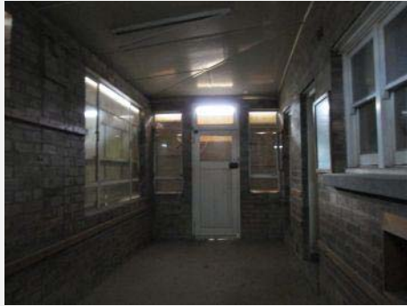
Plate 126: Interior showing room to west end with later addition (right)
