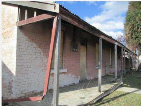
Plate 162: Cottages 7 & 8 south elevation.
