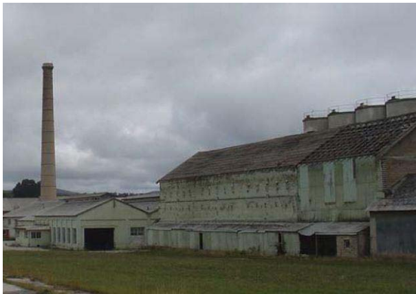
Plate 13: 2013 Cement Store (No.2 Cement Silo) now demolished (Source: Heritage Archival Recording 2013)
