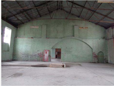
Plate 61: Interior of Western room showing arched openings leading to Central room.
