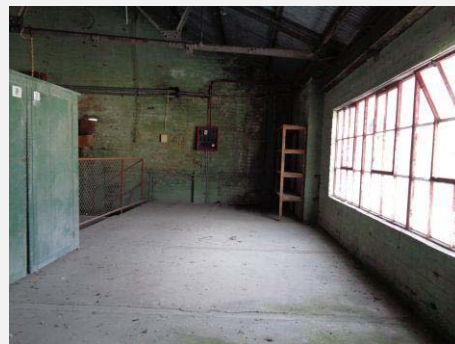
Plate 72: Interior of Eastern room showing detail of mezzanine level.
