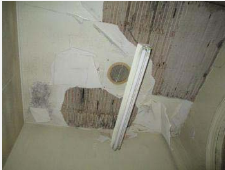
Plate 142: Interior showing lath and plaster ceiling.
