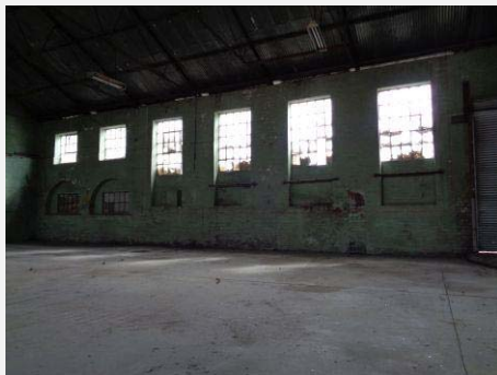
Plate 59: Interior of Western room showing rectilinear openings to north wall.
