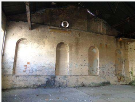
Plate 94: Interior showing Boilermaker's / Blacksmith's Shop.
