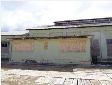
Plate 78: Boilermaker's / Blacksmiths Shop part south elevation.
