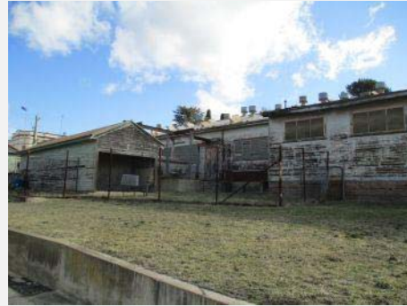
Plate 195: Part east elevation showing garage to the left.
