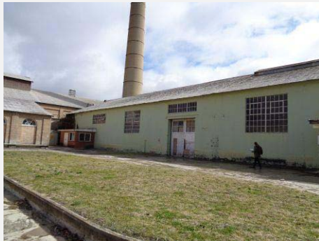
Plate 51: Boilerhouse part south elevation.
