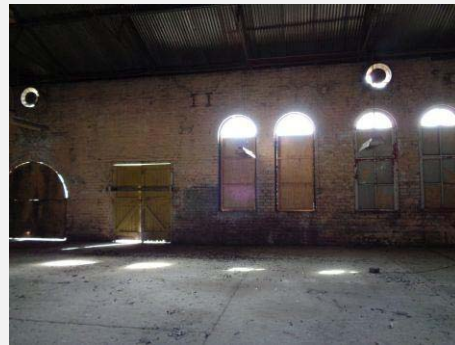
Plate 89: Interior showing Boilermaker's / Blacksmith's Shop.
