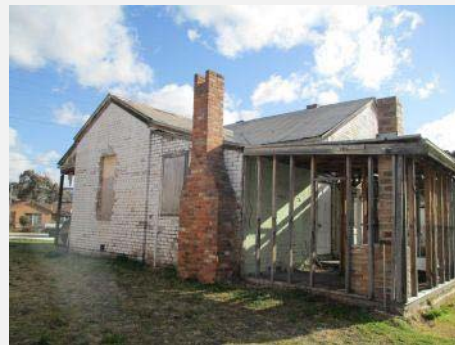
Plate 165: Cottages 9 & 10 east elevation.
