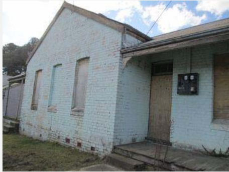
Plate 166: Cottages 11 & 12 south elevation.
