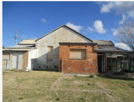
Plate 169: Cottages 13 & 14 north elevation.
