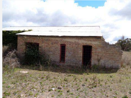
Plate 223: South east view.
