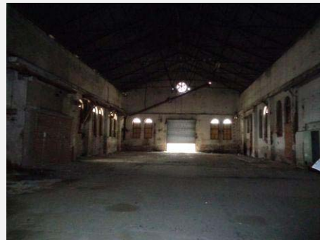
Plate 13: Interior looking north showing roller door to north façade.
