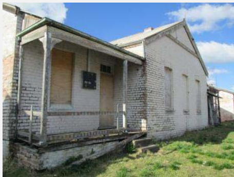
Plate 164: Cottages 9 & 10 south elevation.
