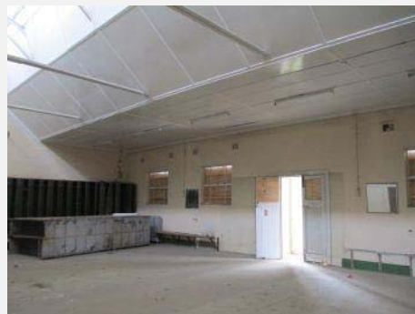
Plate 123: Interior showing entry door and awning windows.
