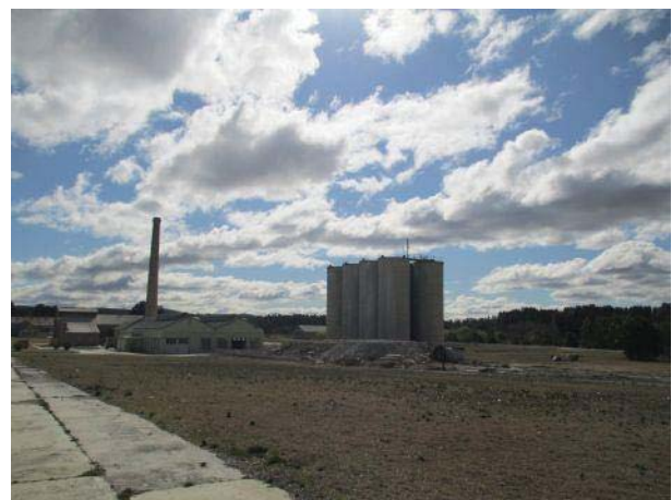
Plate 27: View of Boilermaker's / Blacksmith's shop and Silos looking north west.
