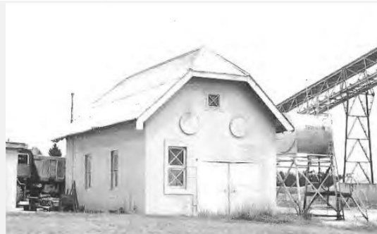
Plate 213: 1993 image of Ambulance Store and Oil tank to right.
