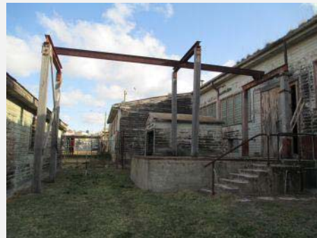
Plate 199: Detail area of east elevation showing brick plinths and gantry.
