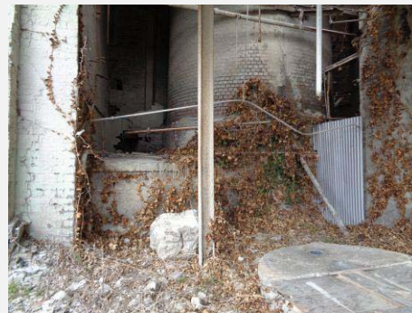
Plate 58: Part north elevation showing base of Chimney.
