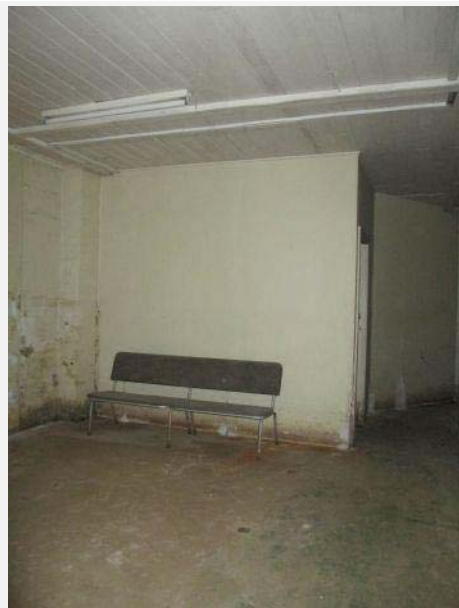
Plate 154: Interior to basement level showing concrete floor and original timber panelled ceiling.
