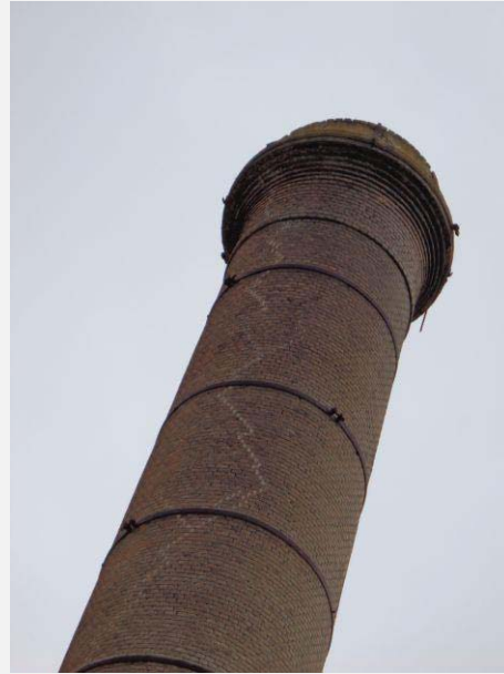
Plate 56: Detail view of Chimney showing iron banding and brick corbelling.
