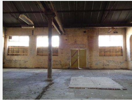
Plate 93: Interior showing Boilermaker's / Blacksmith's Shop.
