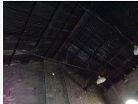
Plate 33: Machinery room showing open steel truss roof.
