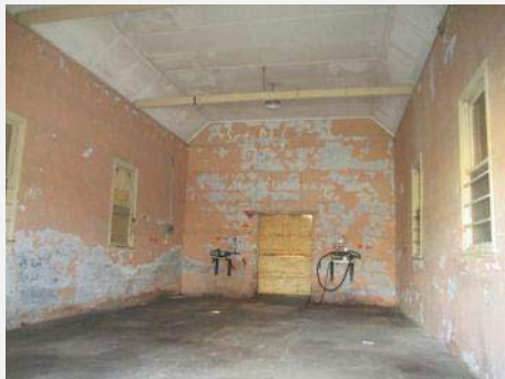
Plate 210: Interior looking west.
