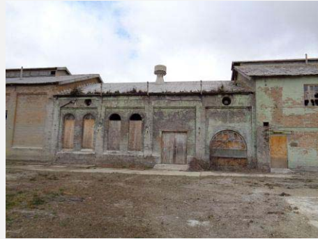
Plate 77: Boilermaker's / Blacksmiths Shop part north elevation.
