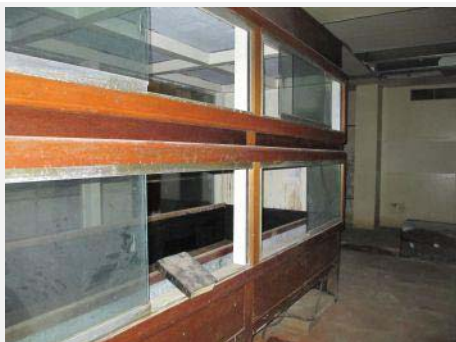
Plate 150: Interior showing timber joinery. This appears to be a prayer room.
