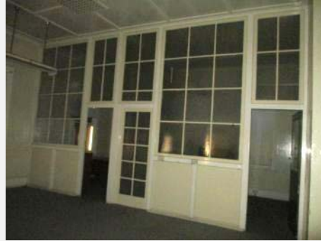
Plate 139: Interior showing intact room with original timber and glass partitions.
