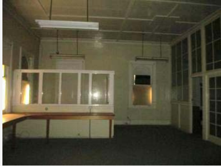
Plate 138: Interior showing intact room with original timber and glass partitions.
