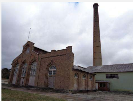
Plate 8: South eastern view showing eastern room.
