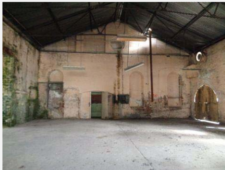
Plate 88: Interior showing Boilermaker's / Blacksmith's Shop.
