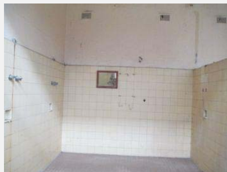
Plate 125: Interior showing typical tiled shower room.
