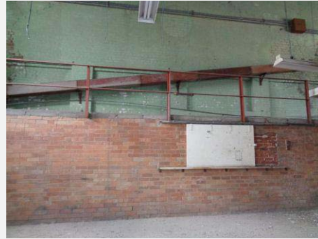
Plate 68: Interior of Eastern room showing ramp to mezzanine level.
