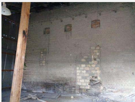
Plate 226: Interior north west room with brick infills.
