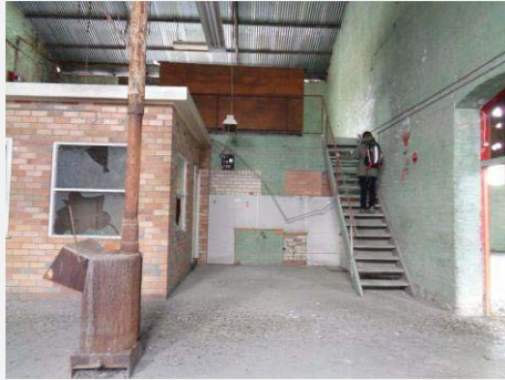
Plate 67: Interior of Eastern room showing mezzanine level, unsympathetic face brick addition.
