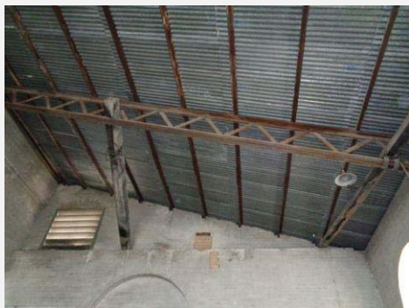
Plate 36: Eastern room showing timber beams insertion to steel truss roof.
