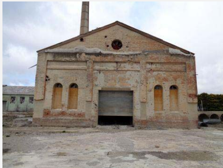
Plate 6: North elevation showing original building.
