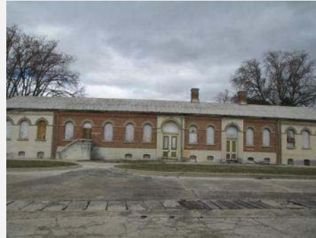
Plate 112: Rail line showing mixture of concrete and timber panels.
