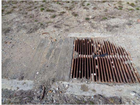
Plate 111: Rail line detail showing timber boarding and metal grate.
