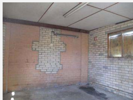
Plate 188: Interior of Store room showing later addition.
