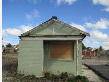
Plate 106: Part west elevation showing original building (left) additions (right with lighter brickwork).
