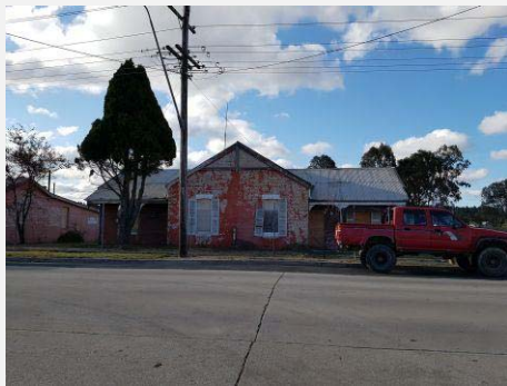
Plate 160: Cottages 5 & 6 south elevation.
