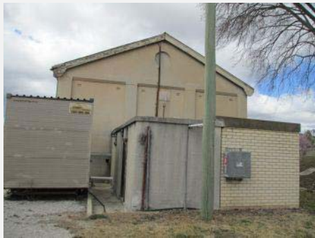
Plate 134: Administration Office west elevation.
