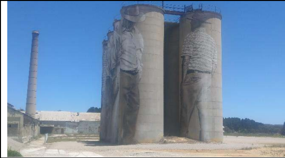
Northern Side of building – fibro on ground
