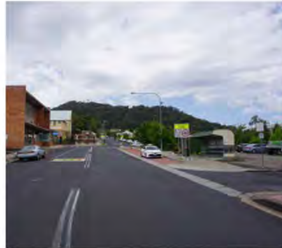
1. View south along Eskbank Street, looking toward the vegetated escarpment east of the Pottery Estate
