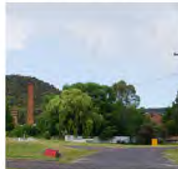
2. Lithgow Valley Colliery & Pottery - present condition
