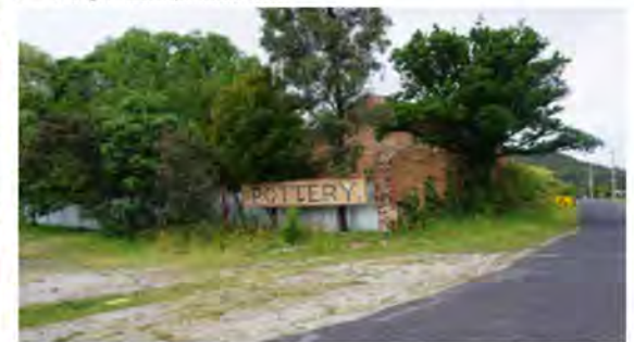
5. The remains of the Lithgow Valley Pottery lack public realm design befitting its historic significance.
