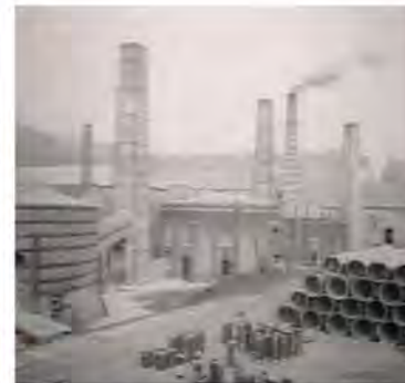
3. Brick and drainpipe works, Lithgow Valley Colliery Co 1906
