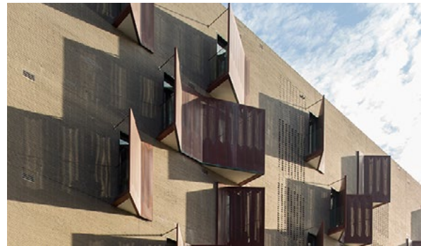
Figure 3-100 Angled privacy screens direct views away from the side boundary. They could also include bay windows
