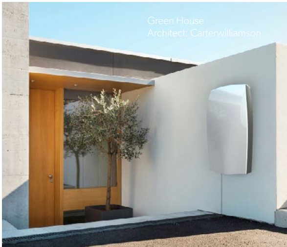
Figure 3-134 Battery storage saves energy generated during the day for use in the evening
