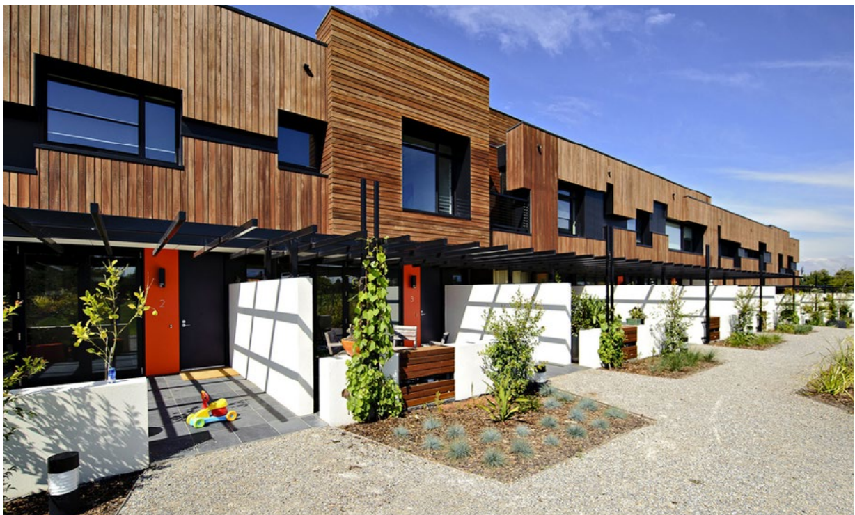
Figure 1-25 Example of multi-dwelling housing with pedestrian street access
