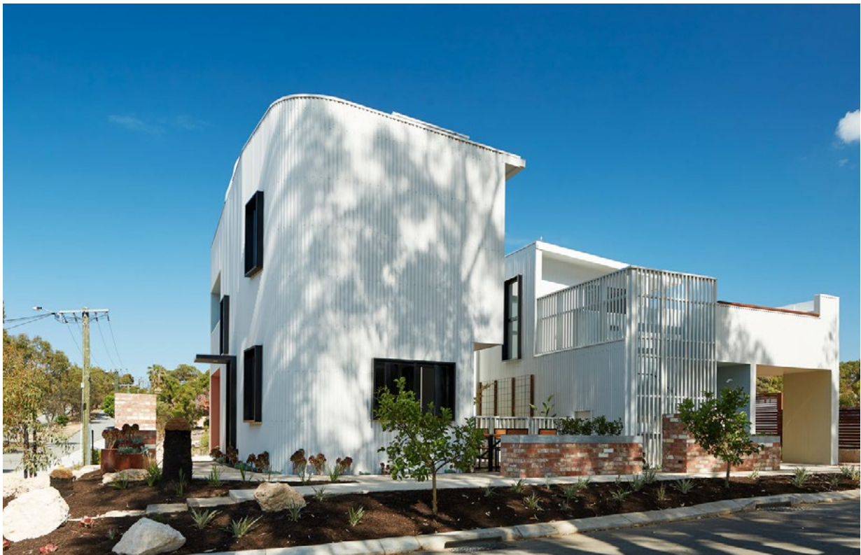
Figure 2-30 Manor House - 3 dwellings
