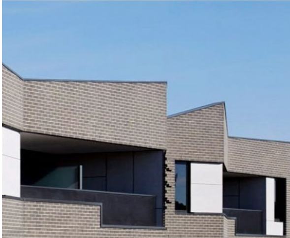
Figure 3-115 Silhouette created by parapet
