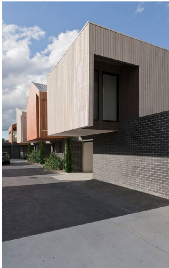
Figure 3-108 A poor acoustic outcome is achieved when driveways are in close proximity to bedrooms and living rooms, and driveways are hard paved reverberating sound.
