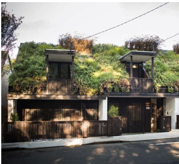
Figure 3-47 Green roof on terraces
