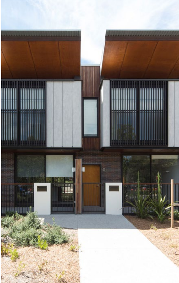
Figure 3-109 Living rooms setback from main circulation spaces by large landscape setback provides privacy
