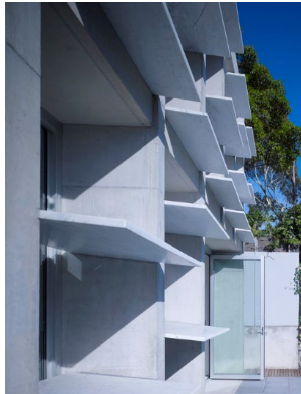
Figure 3-133 Light shelves can reflect sunlight deeper into rooms and provide shade from summer sun
