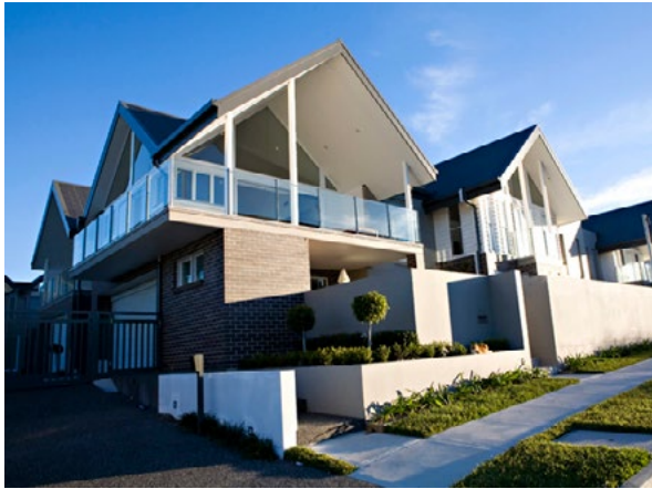
Figure 3-116 Roof form expressed
