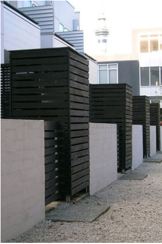
Figure 3-143 Bin areas fronting the street can be designed and incorporated into the building or landscape elements
