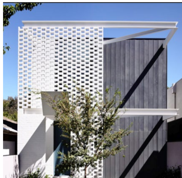
Figure 3-101 Privacy screens are integrated into the facade and provide part of the architectural expression
