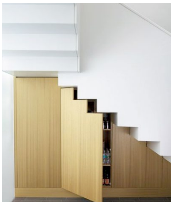
Figure 3-93 Storage space under stairs
