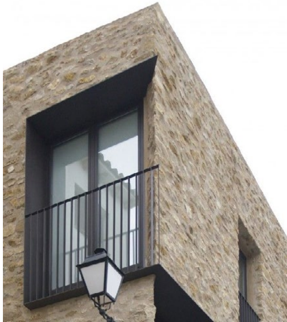
Figure 3-124 Contrast texture with sharply defined openings and fine steel balustrades
