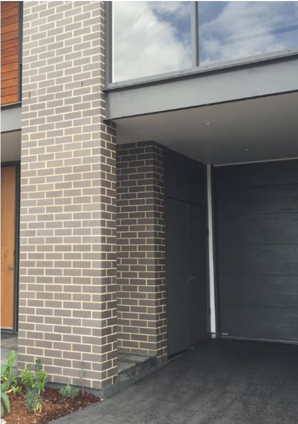
Figure 3-142 Provide bin areas that are screened and incorporated into the landscape or building design
