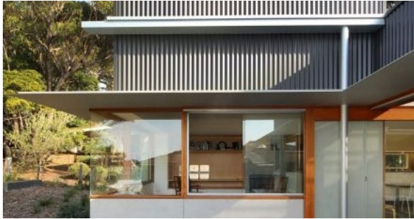
Figure 3-123 Awnings provide shelter and add articulation
