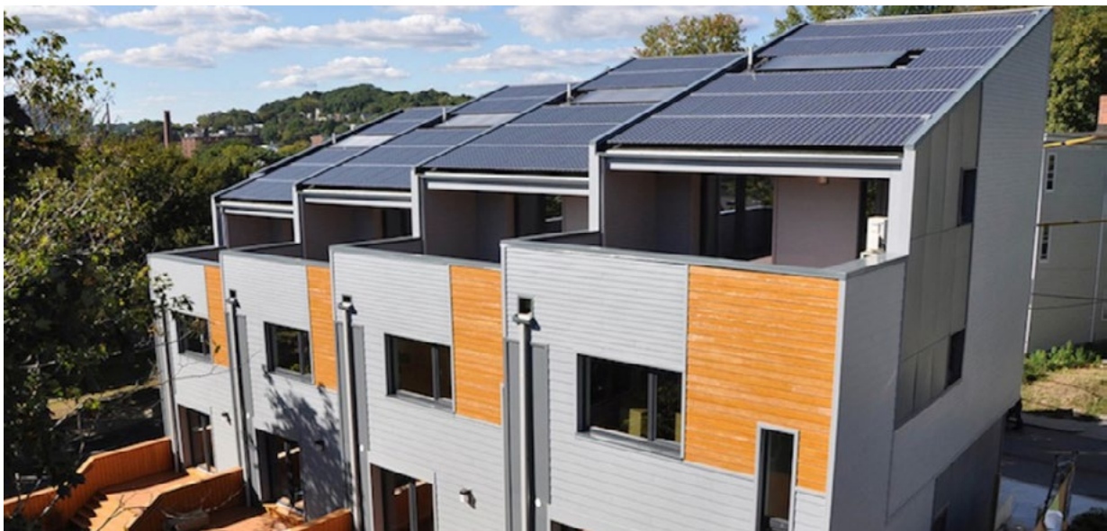
Figure 3-132 Roof mounted photovoltaics should be integrated into the design of the dwelling
