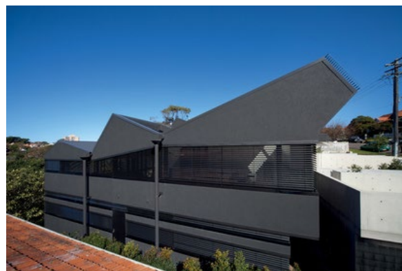
Figure 3-114 Interesting roof forms and integration of privacy and sun control devices to overall building design
