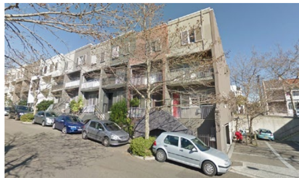
Figure 3-64 Reduce visual impact of basement entries by reducing the scale of the opening
