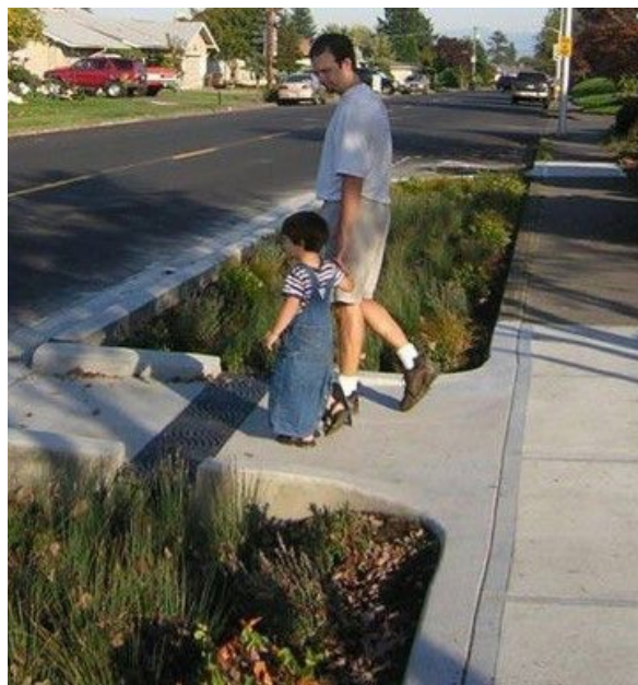
Figure 4-155 Rain gardens treat stormwater from the streets
