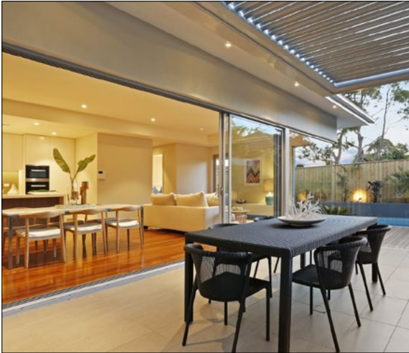
Figure 3-148 A universally designed dwelling provides step free door transitions and level flooring to reduce trip hazards
