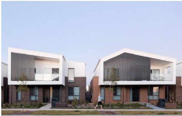
Figure 3-125 The use of screens provides privacy to balconies
