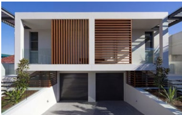
Figure 3-107 Privacy screens can be an integral part of the articulation. Changing the pattern and direction of the screen adds visual interest and asymmetry to the facade.
