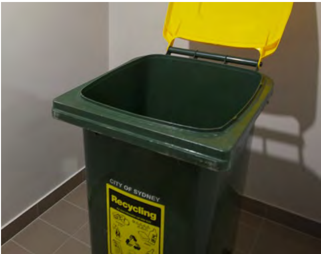
Figure 4W.5 Waste and recycling areas should allow for sufficient space to manoeuvre bins and sort waste for recycling
