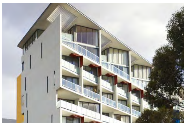
Figure 4B.5 Natural cross ventilation is facilitated by limited apartment depths and use of dual aspect apartments
