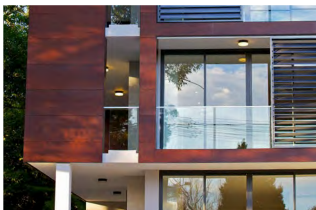
Figure 4B.6 Natural ventilation is further enhanced by using generous window and door openings
