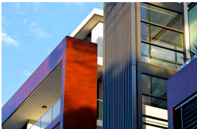
Figure 4M.3 Building articulation such as balconies and deeper window reveals provide visual interest to the facade
