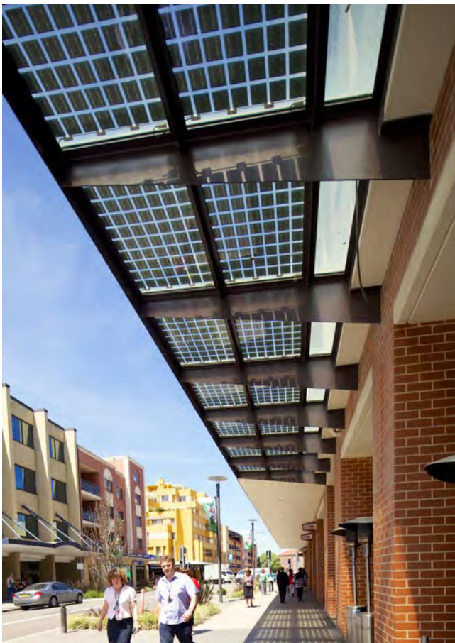
Figure 4U.5 Environmental technology, integrated into the overall design, adds to the sustainable performance of buildings
