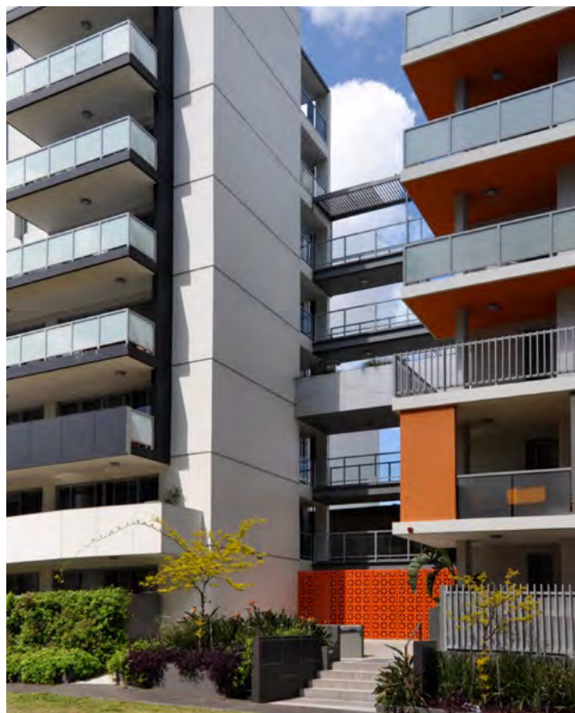
Figure 3G.2 Breaks between buildings, colour and landscaping can be combined to help identify building entries
