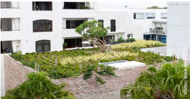
Figure 4P.3 Roof top planting requires careful plant selection and an understanding of the local climate conditions
