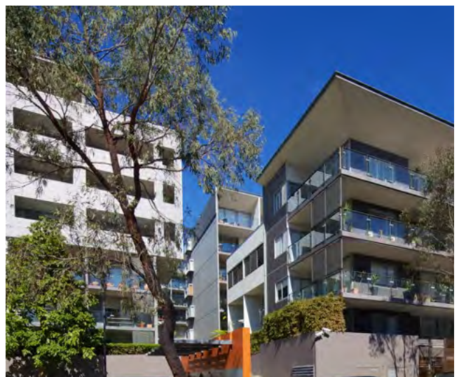
Figure 2H.4 Side and rear setbacks vary according to the building context and type. In urban areas, setbacks are often guided by minimum building separation requirements
