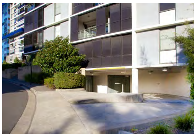
Figure 3H.2 Clear sightlines help to keep pedestrians safe. Locating entries to car parks at the lowest level of the site reduces ramp length
