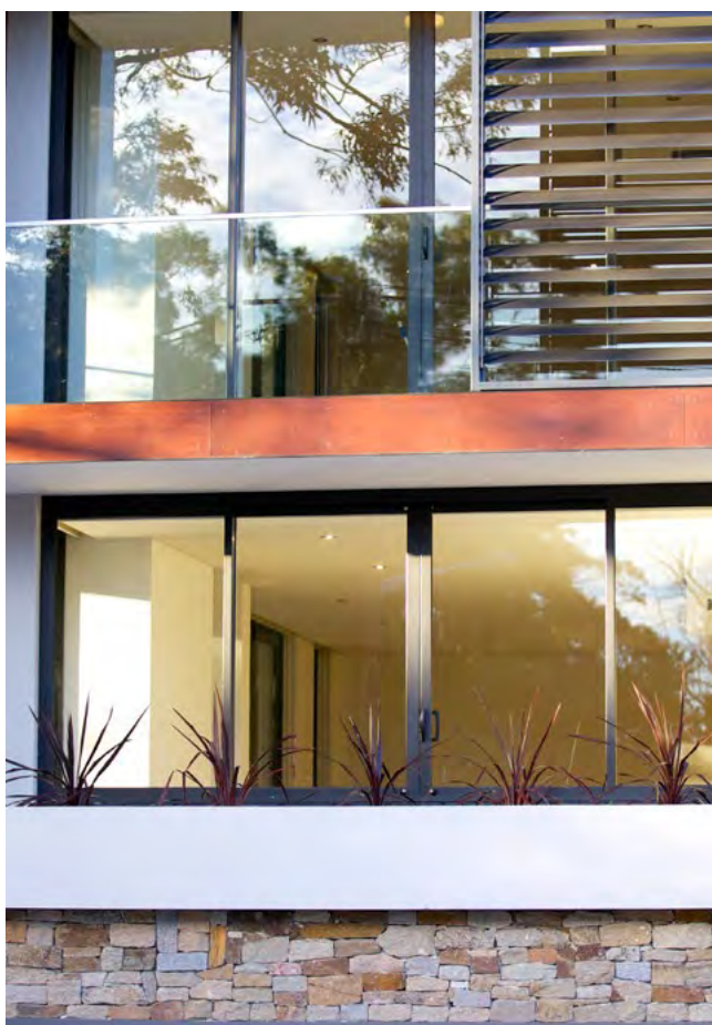
Figure 4H.5 In addition to mindful siting and orientation of the building, acoustic seals and double or triple glazing are effective methods to further reduce noise transmission
