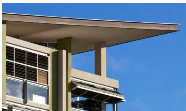
Figure 4N.3 Solar access to apartments can be maximised by tilting roof elements towards the north
