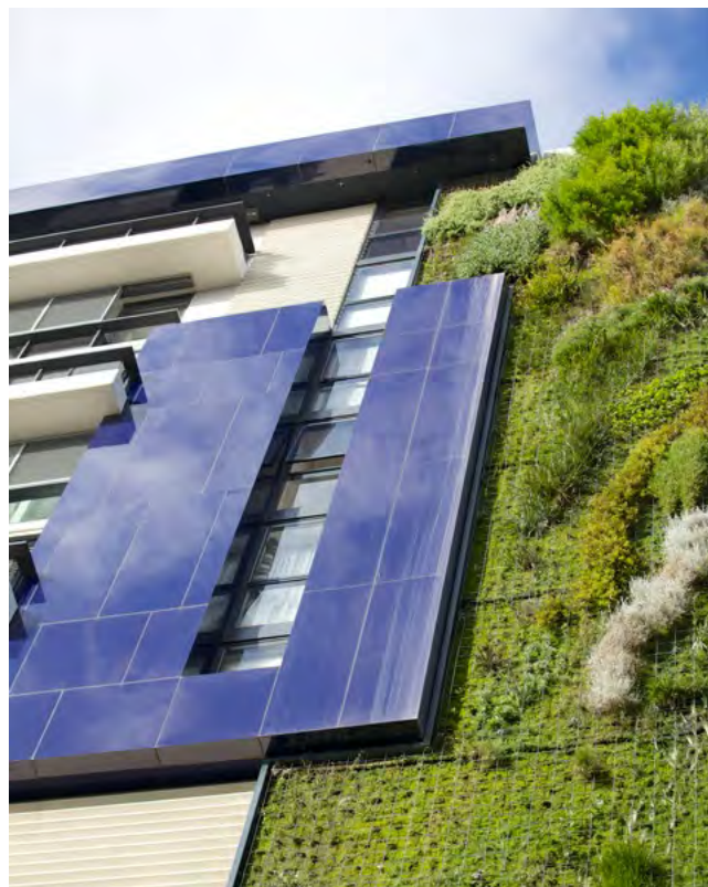
Figure 4P.1 Green walls and facades make positive contributions to the environment and to urban amenity more generally. They can also improve the sustainability performance of a building
