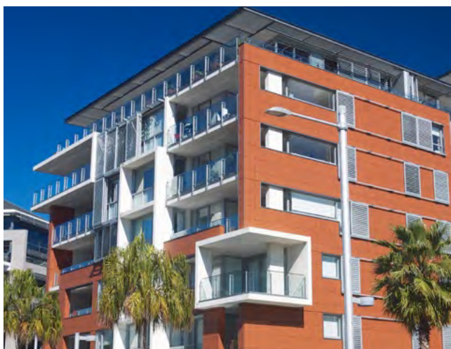
Figure 4M.4 The terracotta tile cladding used on this building contrasts with the white framed balconies and roof line, adding visual interest
