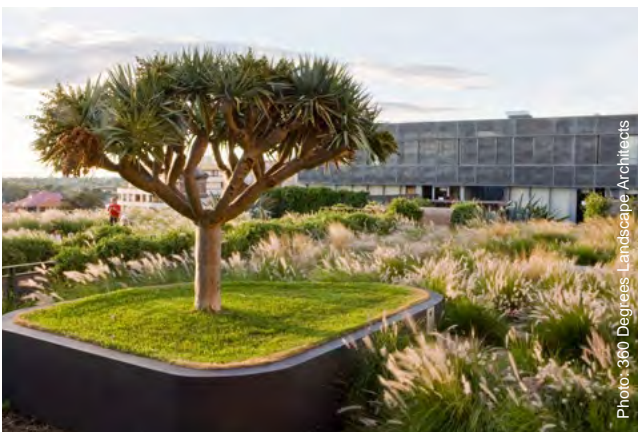
Figure 4P.4 Methods for planting on structures include raised planters and a mix of shallow and deep profile garden beds
