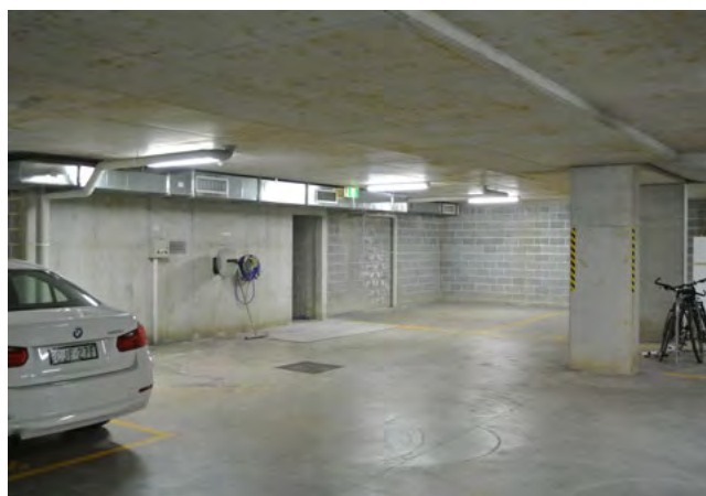
Figure 3J.9 Car wash bays can be accessed without crossing car parking spaces
