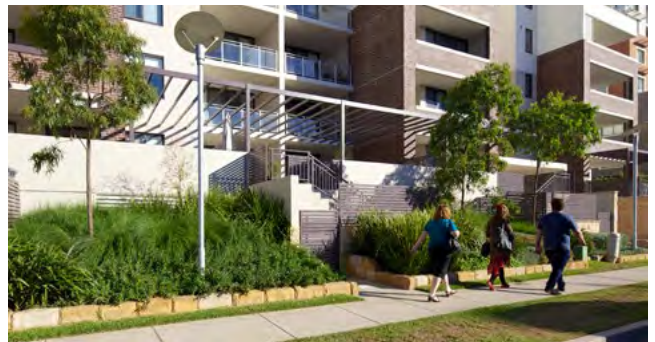
Figure 2G.2 This example provides a landscaped setback which contributes to the residential character of the street
