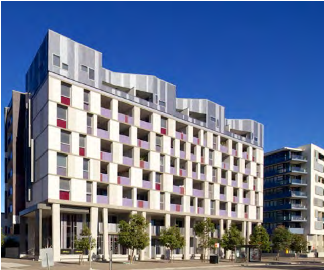
Figure 4N.4 The composition of this roof form creates a skyline silhouette and contributes to the identity and character of the area
