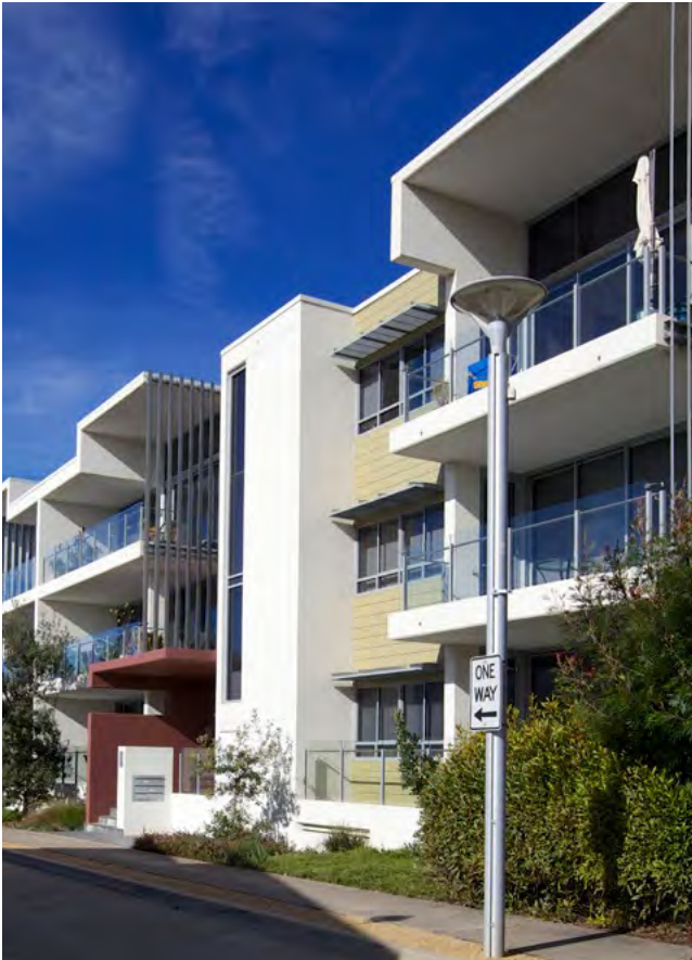
Figure 4X.3 Roof overhangs, hoods and drip lines protect walls from the elements (rain, sun and wind) reducing maintenance costs
