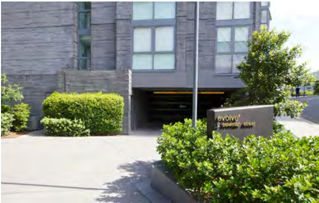
Figure 3H.4 The visual impact of vehicle entries can be minimised by an offset alignment of the driveway and screen planting
