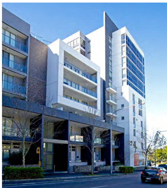
Figure 2E.3 Building depth dimensions should include articulation such as projecting balconies, gallery access, overhangs, blades and other architectural features
