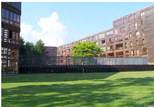
Figure 3J.6 Natural ventilation to the underground car park is integrated into the landscape design of this development
