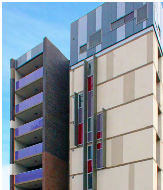
Figure 4M.1 Thoughtful modulation of the facade reduces the perceived depth and bulk of a building
