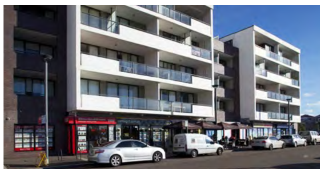
Figure 3J.1 This development provides green open space on top of the car park structure (top photo). The ground level facing the street is 'wrapped' with retail and commercial uses (bottom photo)
