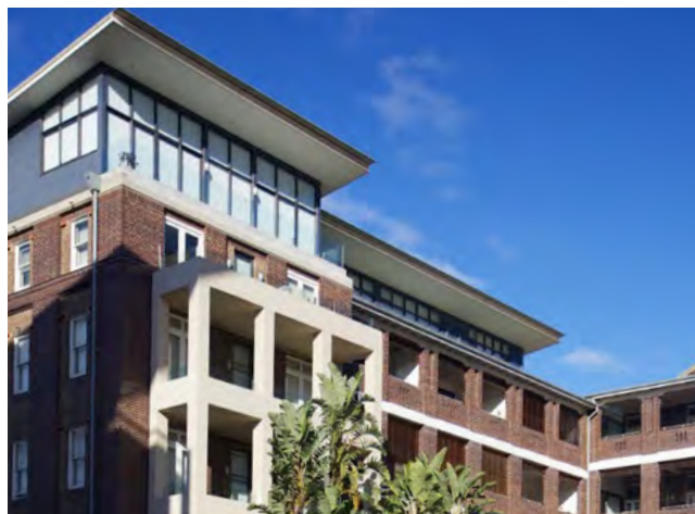
Figure 4R.1 Modern materials can be used if their proportions and details suit the building and context, and allow for interpretation of old and new building elements
