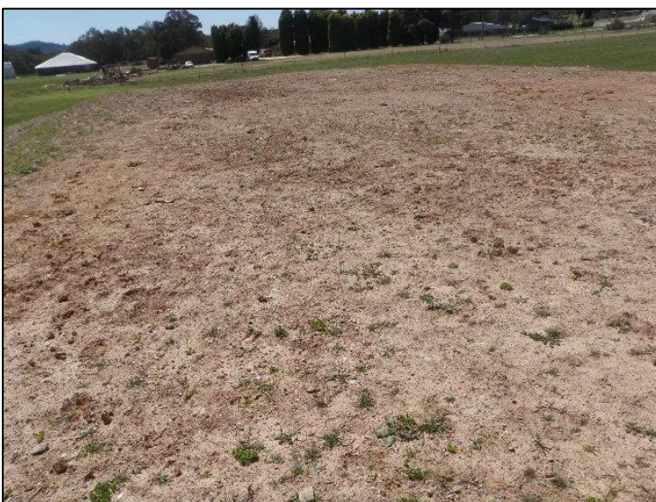
Looking north across imported fill pad
