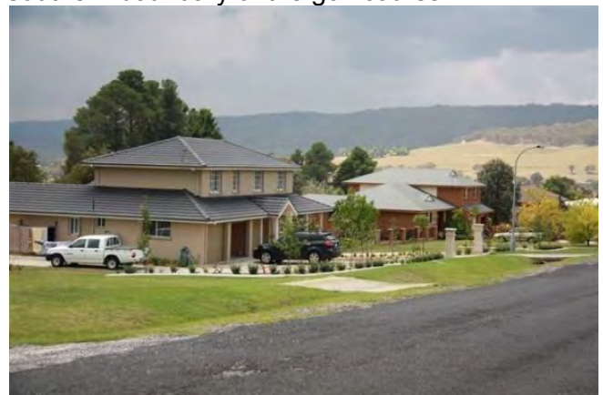
An example of residences in Marrangaroo Fields Estate, adjoining the golf course.
