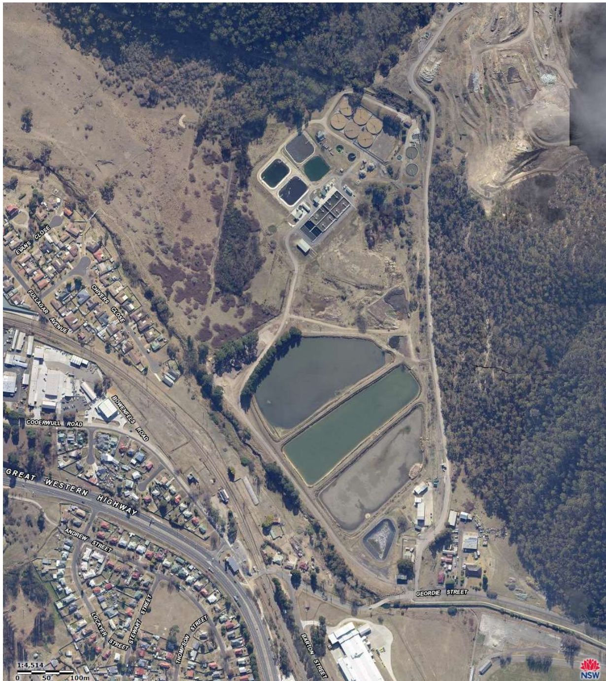
Figure 1 - Recent satellite imagery of the Lithgow Sewage Treatment Plant
