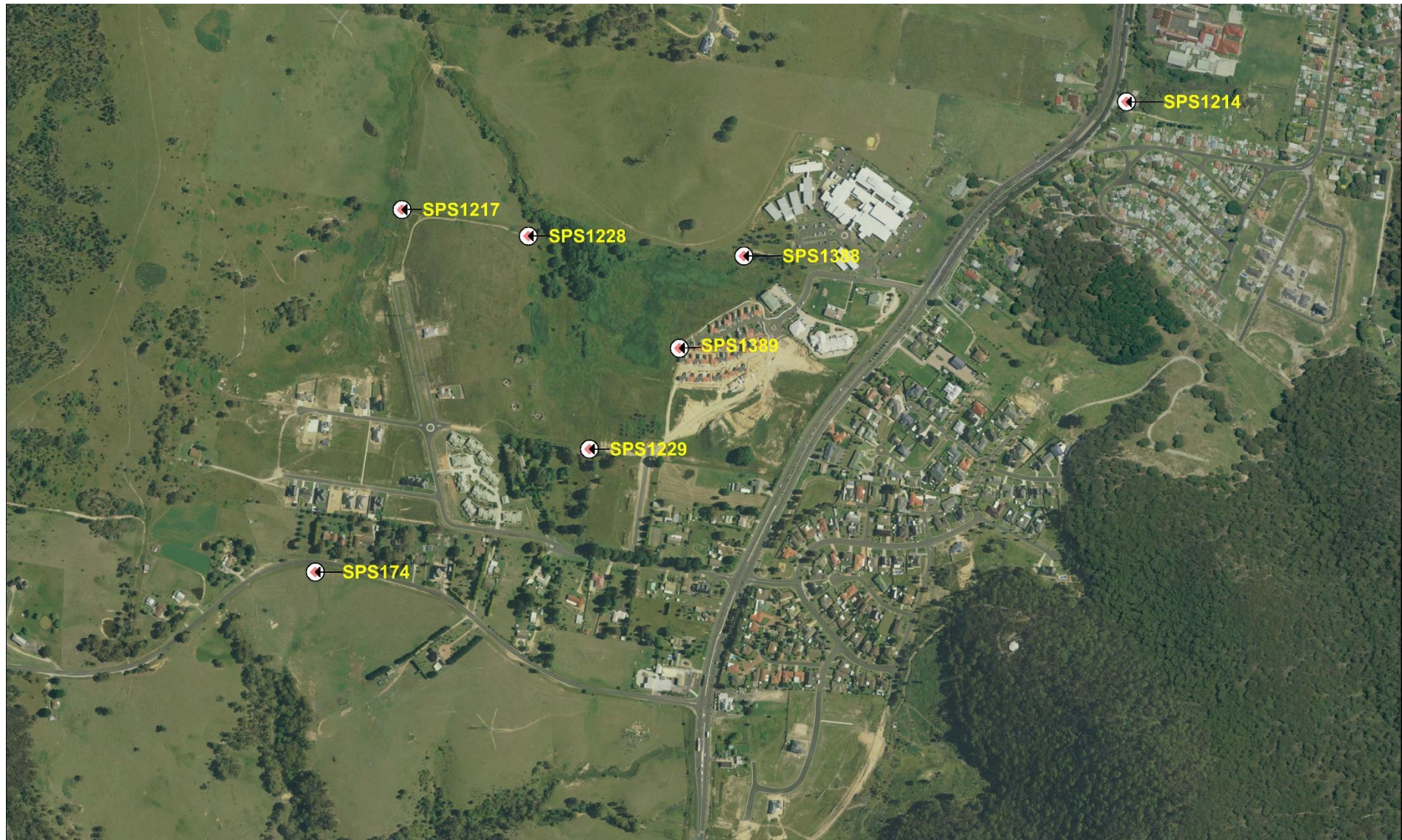
Figure 9 - South Littleton & Bowenfels pump stations
