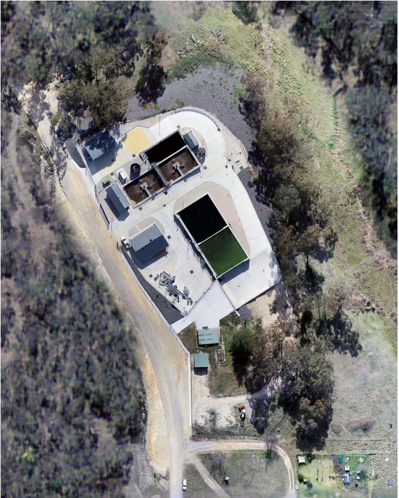
Figure 1 - Recent satellite imagery of the Portland Sewage Treatment Plant
