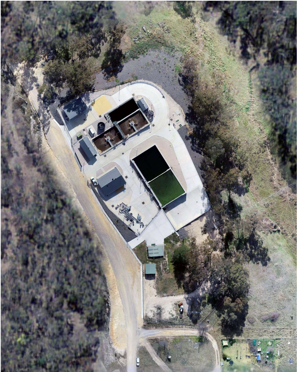
Figure 1 - Recent satellite imagery of the Portland Sewage Treatment Plant
