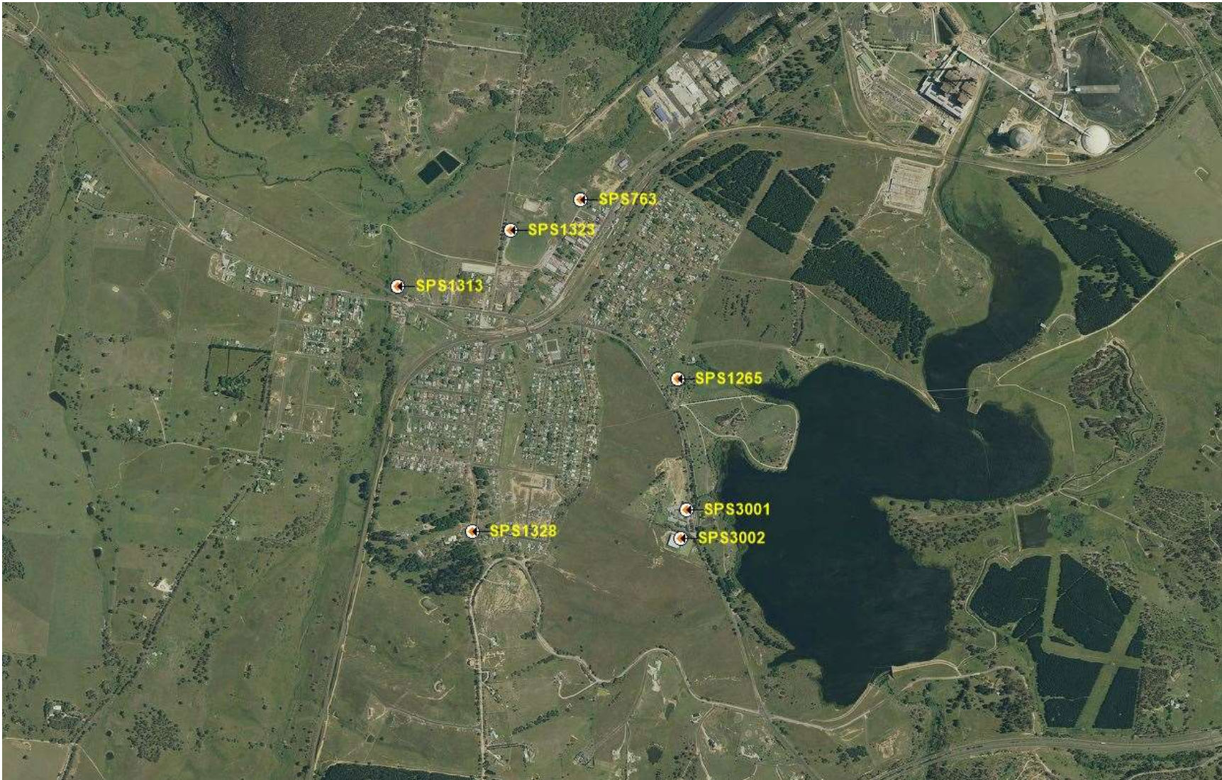
Figure 4 - Wallerawang pump stations
