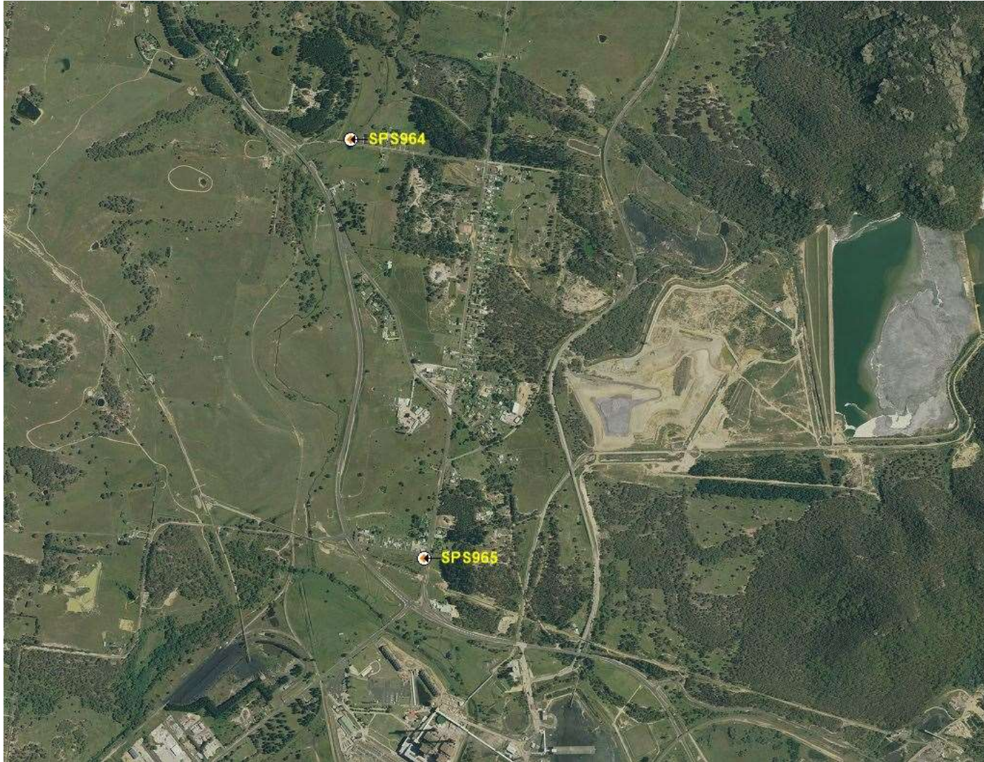
Figure 6 – Lidsdale Pump Stations
