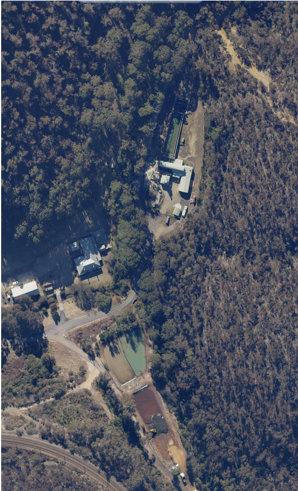
Figure 1 - Recent satellite imagery of the Oakey Park Water Treatment Plant
