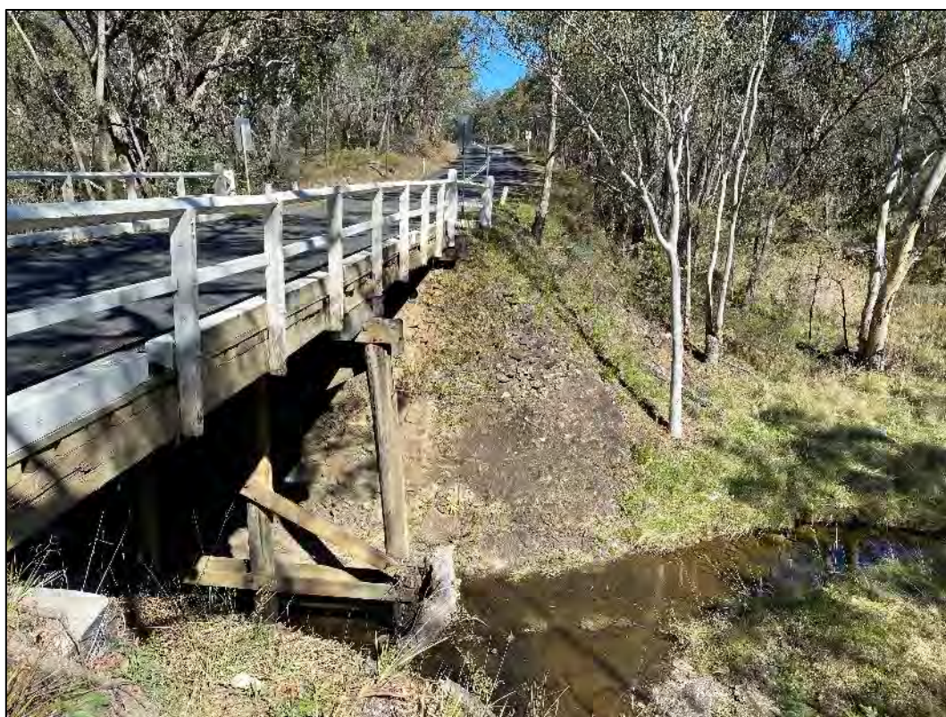
Plate 3: Looking west across the built up creek bank and wooden piers for Airly Creek bridge.
