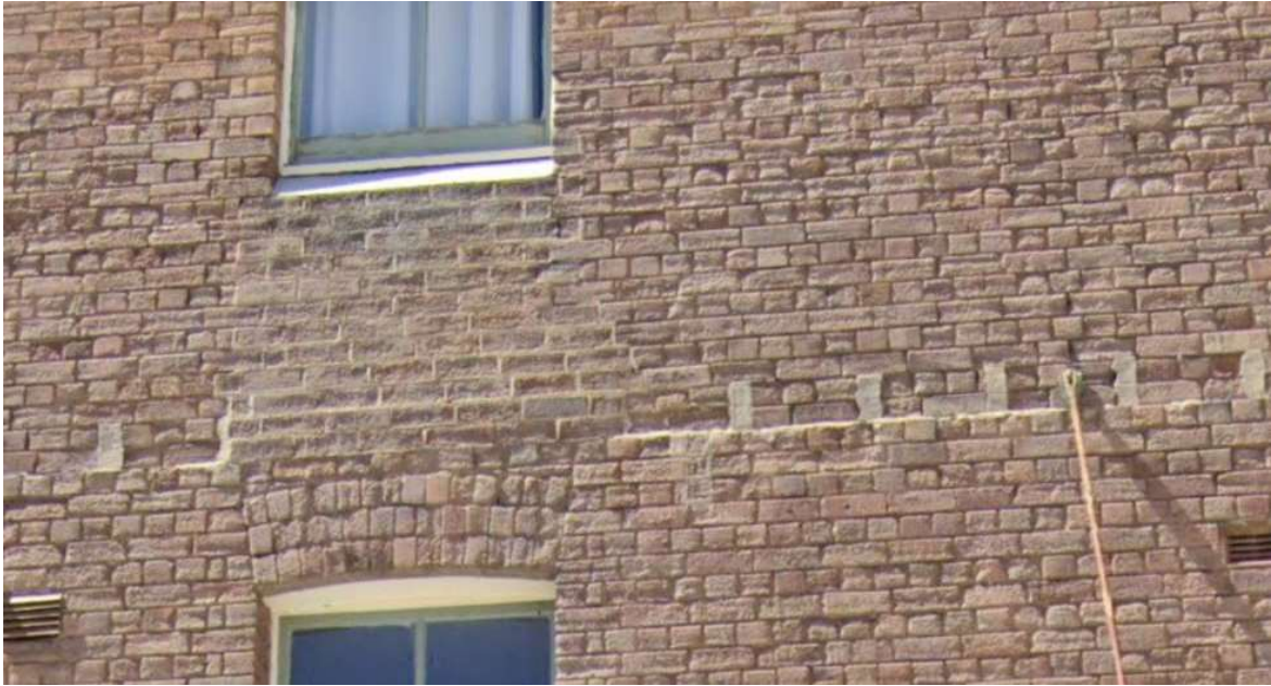
Figure 34: View of brickwork where verandahs were removed
