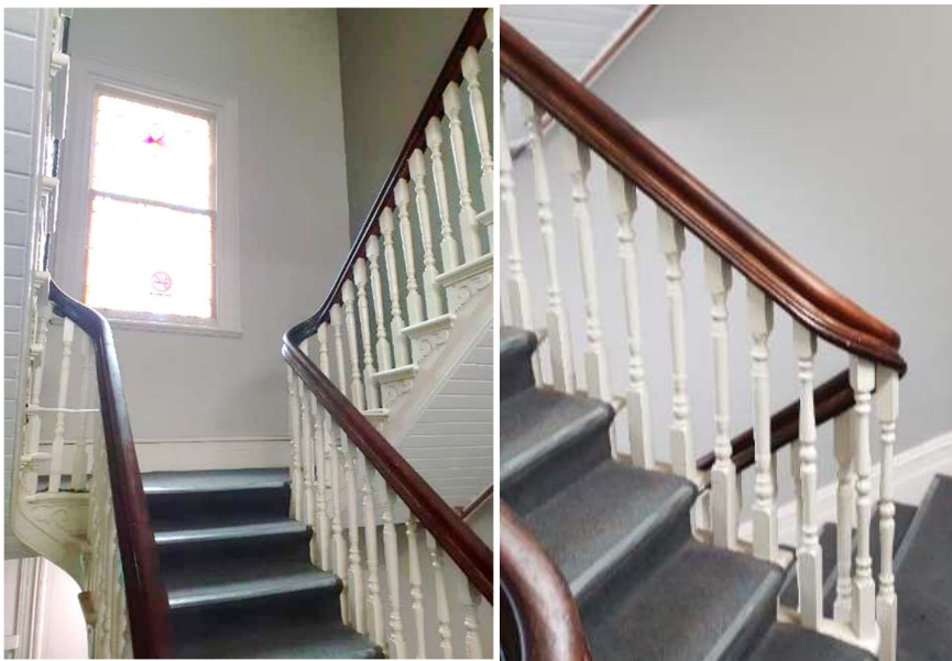
Figure 43: Views of original staircase with some balusters being mismatching replacements
