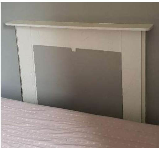
Figure 41: Possibly original fireplace mantelpiece, with missing detail.
