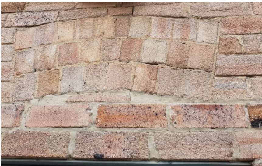
Figure 34: View of brickwork where verandahs were removed
