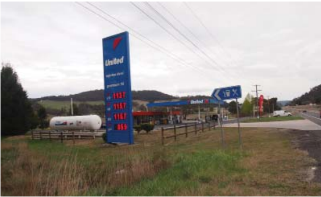
Highway service station
