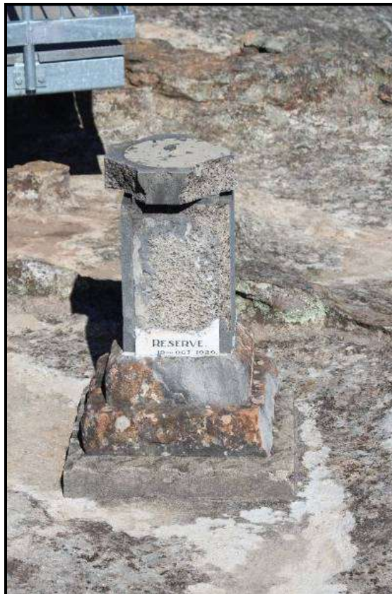
Remains of the plinth (the Padley Memorial Direction Dial) at Hassans Walls Lookout
